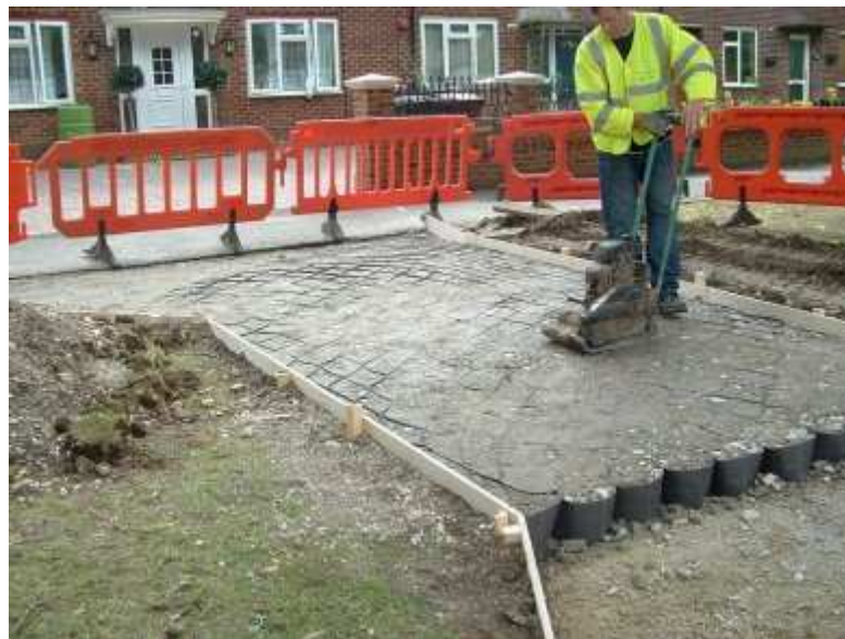
Fig 1. Cellular confinement system
