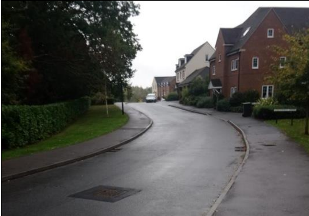
Figure 6-2: Pedestrian provision on Greenhurst Drive
