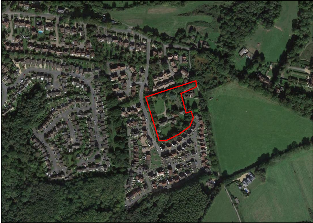
Figure 2-1: Site Location (courtesy of Google Maps)
