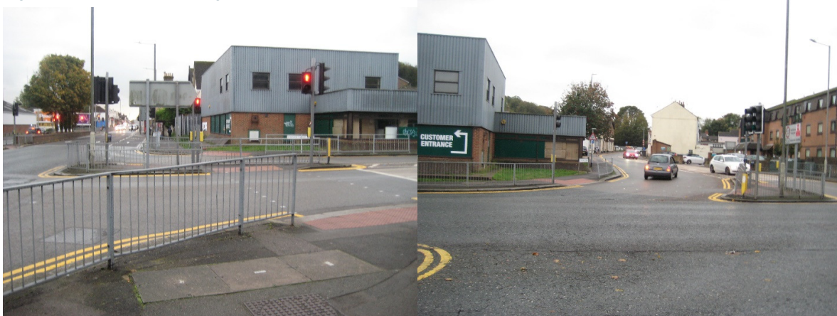
Figures 2.5 & 2.6 – Looking southeast & southwest at the London Rd/Coombe Valley Rd junction
