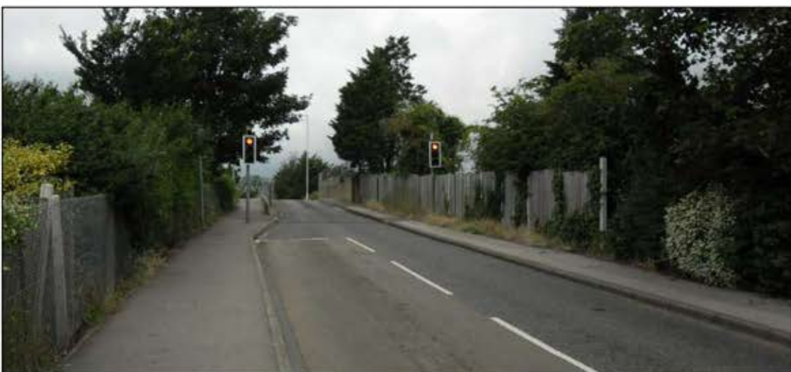
View west along Quinton Road towards single file signals over rail bridge
