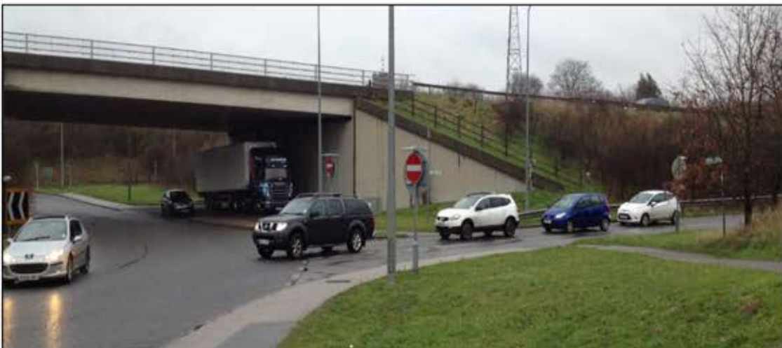
View looking towards southbound off slip at Bobbing junction
