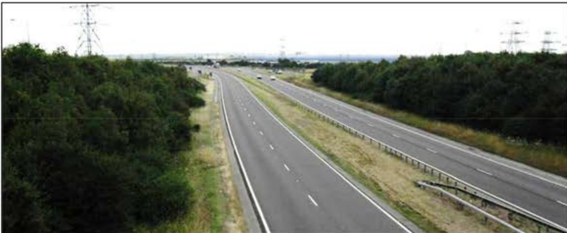
View looking north along the A249 from the Grovehurst Road junction
