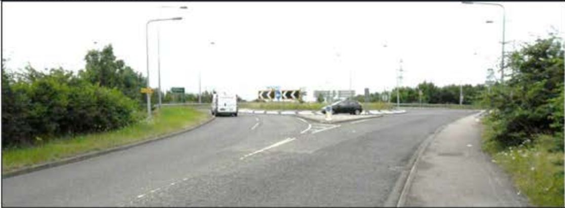
View looking south towards the north roundabout from the B2005 Grovehurst Road
