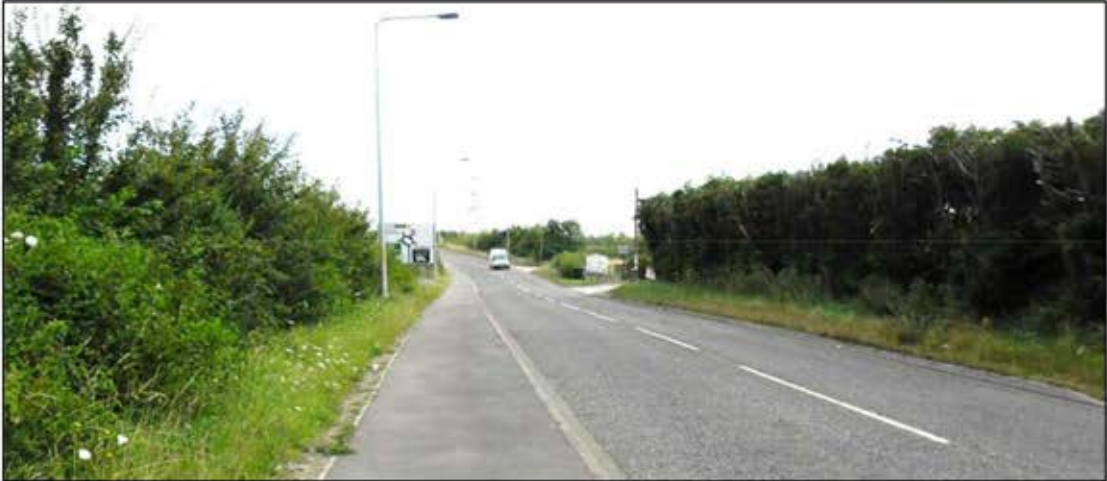
View north along the B2005 Grovehurst Road on the approach to the A249 junction
