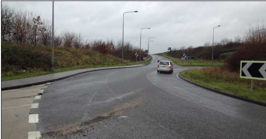
View looking towards southbound on slip at Bobbing junction
