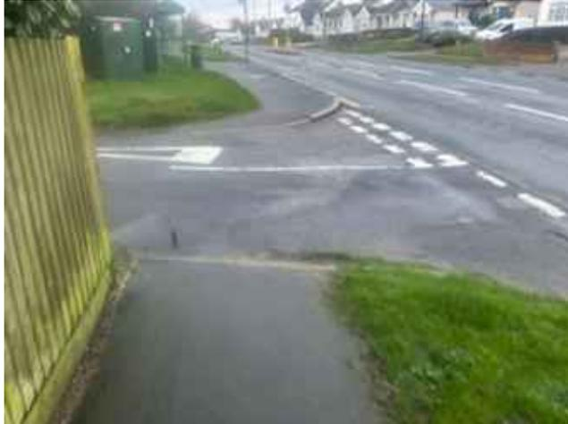
Figure 1: No tactile paving at pedestrian crossing point.
