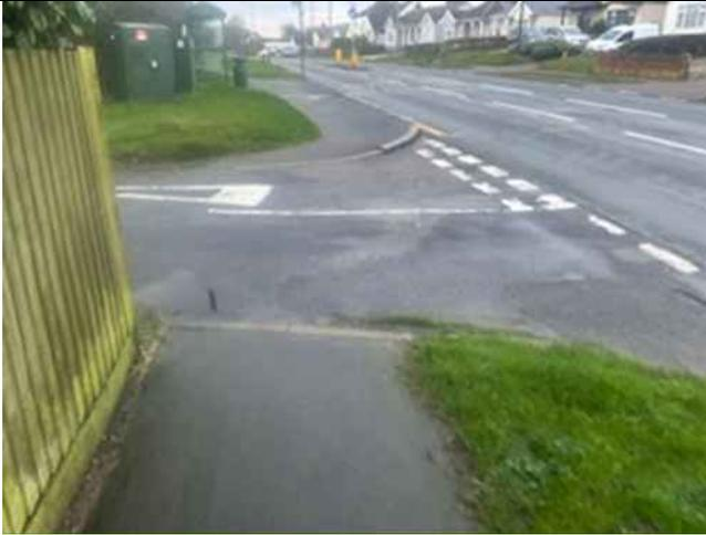
**Figure 3:** Fencing restricting visibility at crossing point.
