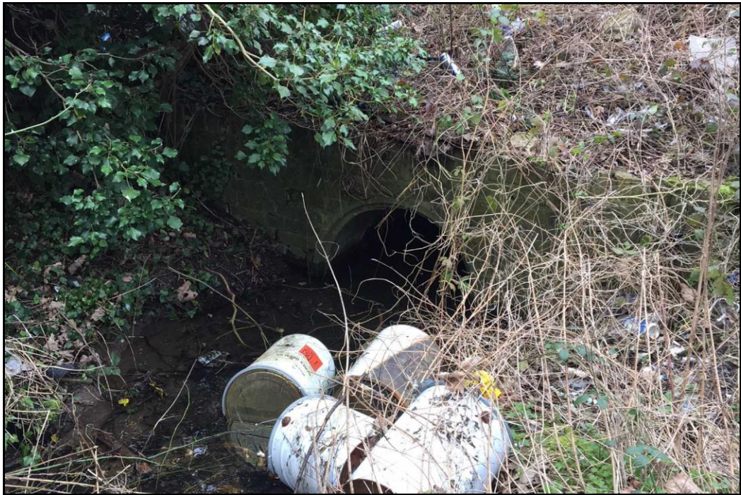
Figure 6. Concrete pipe under Old Ferry Road.
