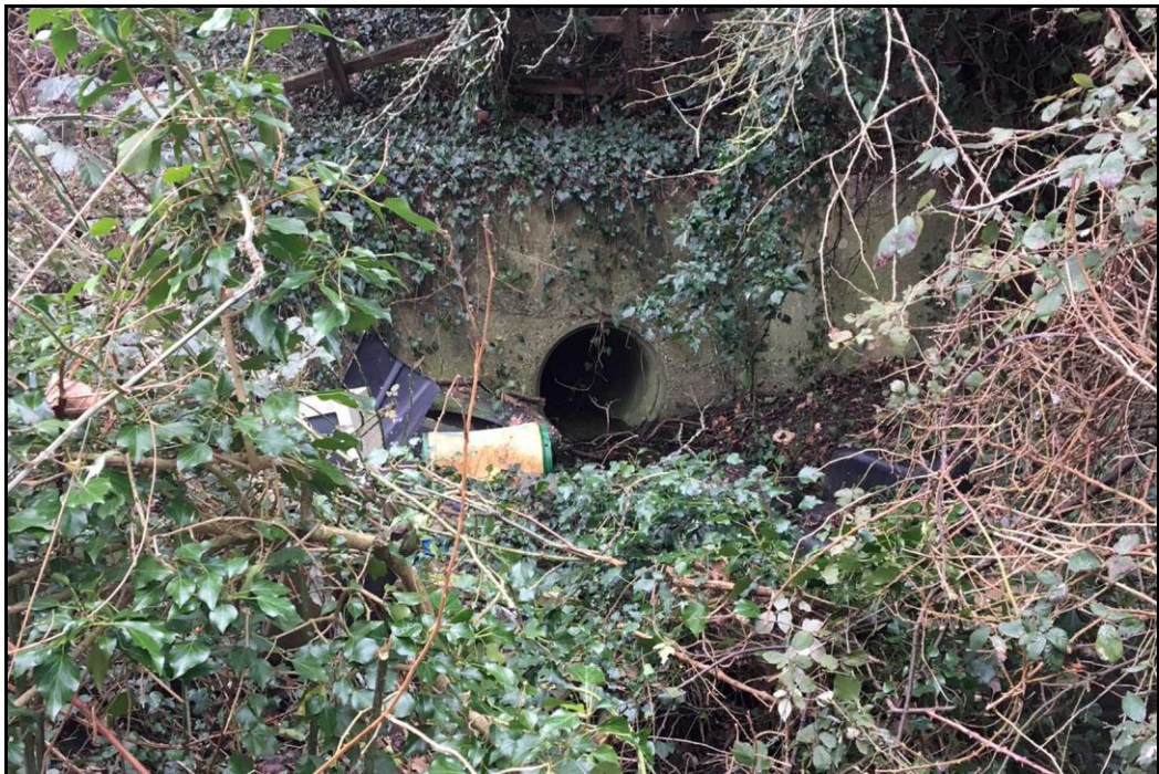
Figure 7. Concrete pipe under Sheppey Way.
