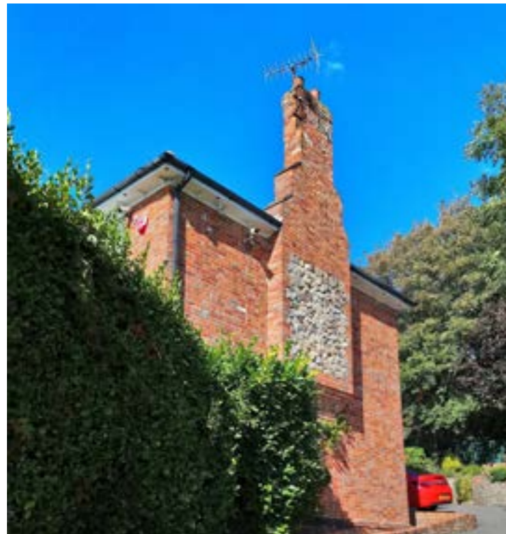
East elevation (no windows) facing the site
