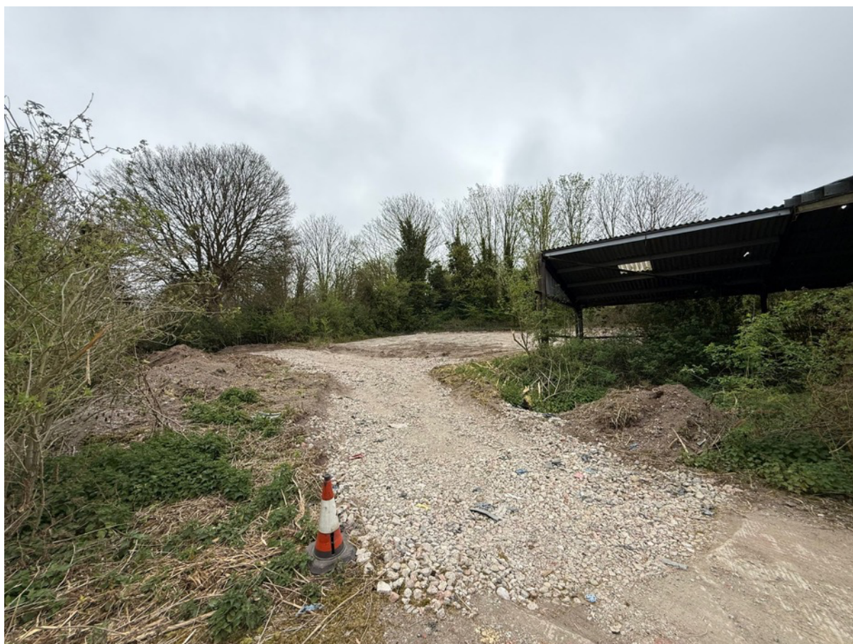
Image shows track created for access and historic position of JK2 and the Bund.
