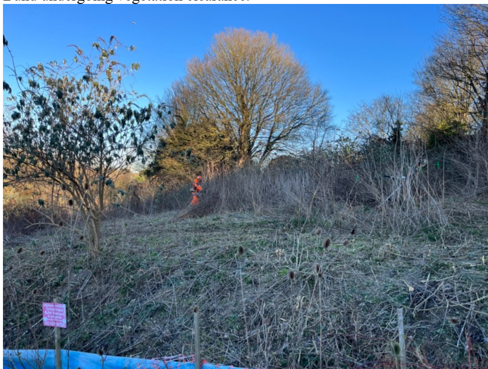
Bund undergoing vegetation clearance.
