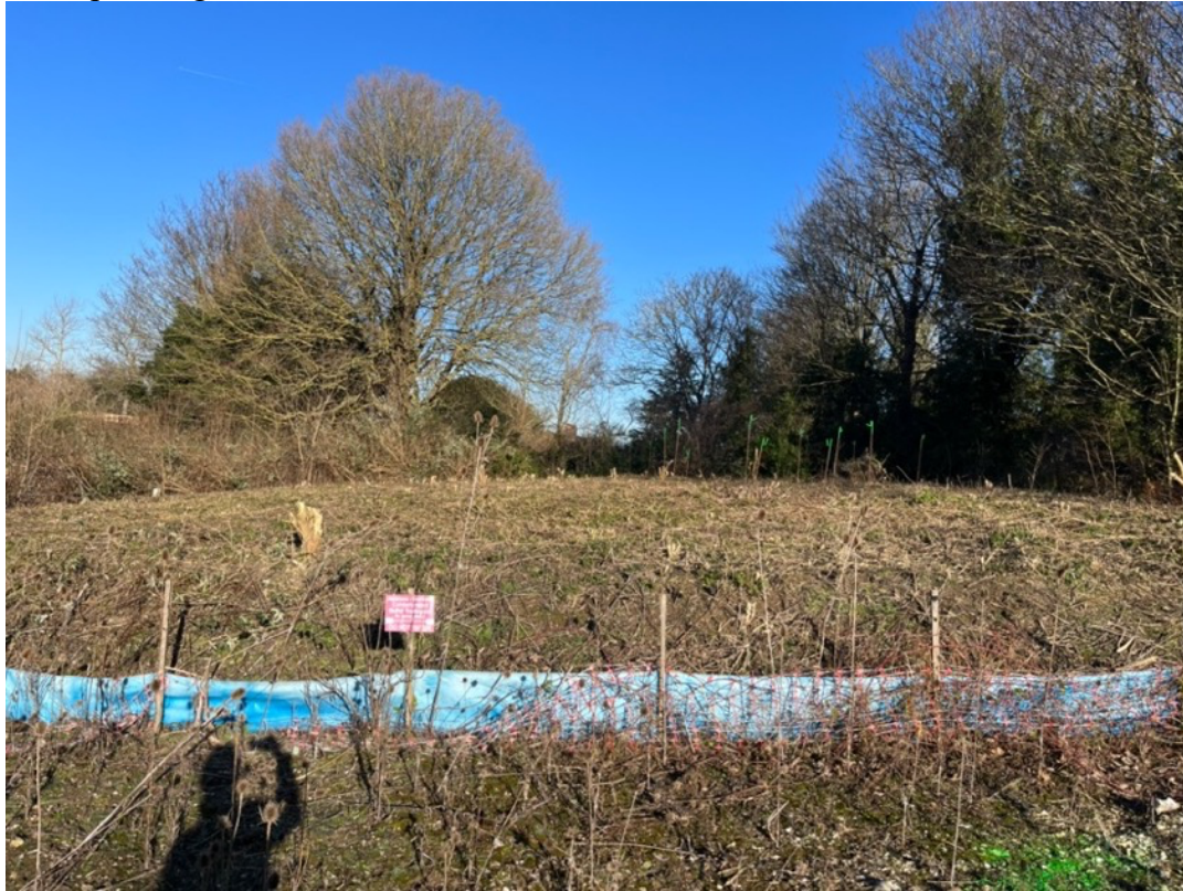
Bund post vegetation clearance.
