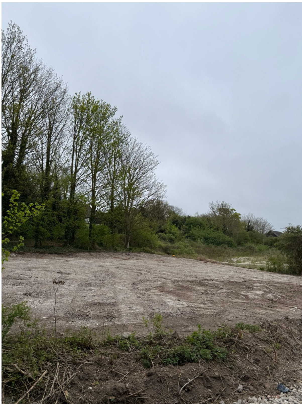
Looking south at the cleared location on completion of works.
