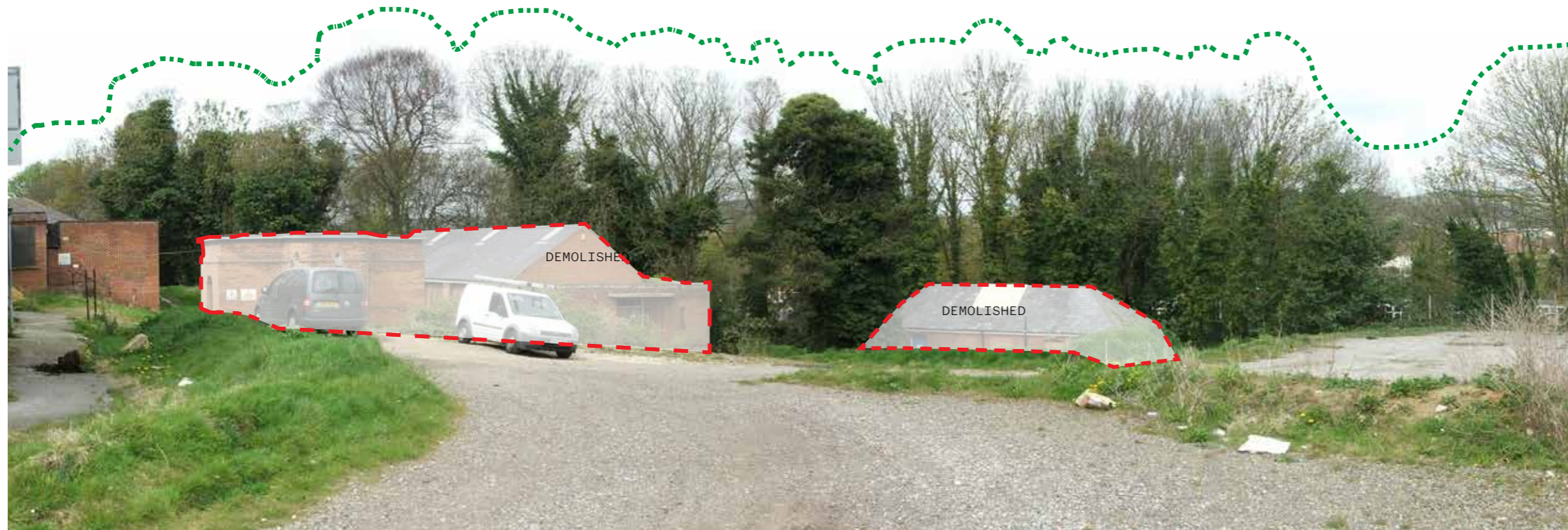
C. View looking at rear of the site showing the now demolished outbuildings, steeply changing levels over the site, hard-standing areas and dense mature trees at the boundary of the site.
