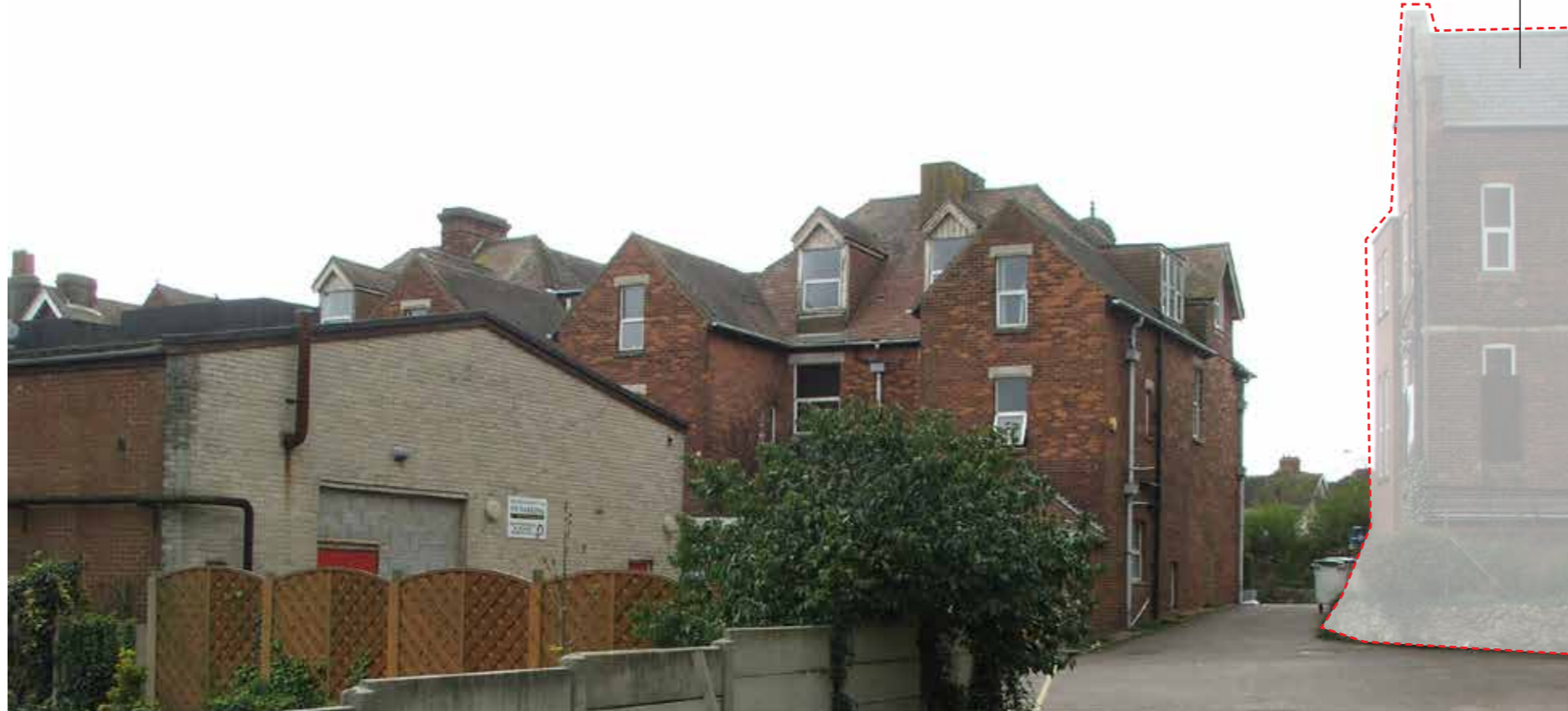
D. View from the former tennis court looking towards the front of the site and the existing right of way access.
