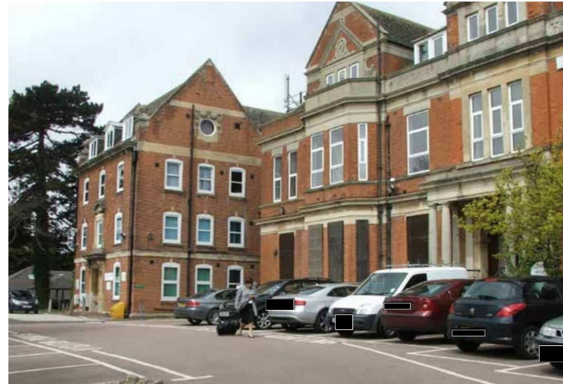
B. View from main access looking at existing car park and main Royal Victoria Hospital building.
