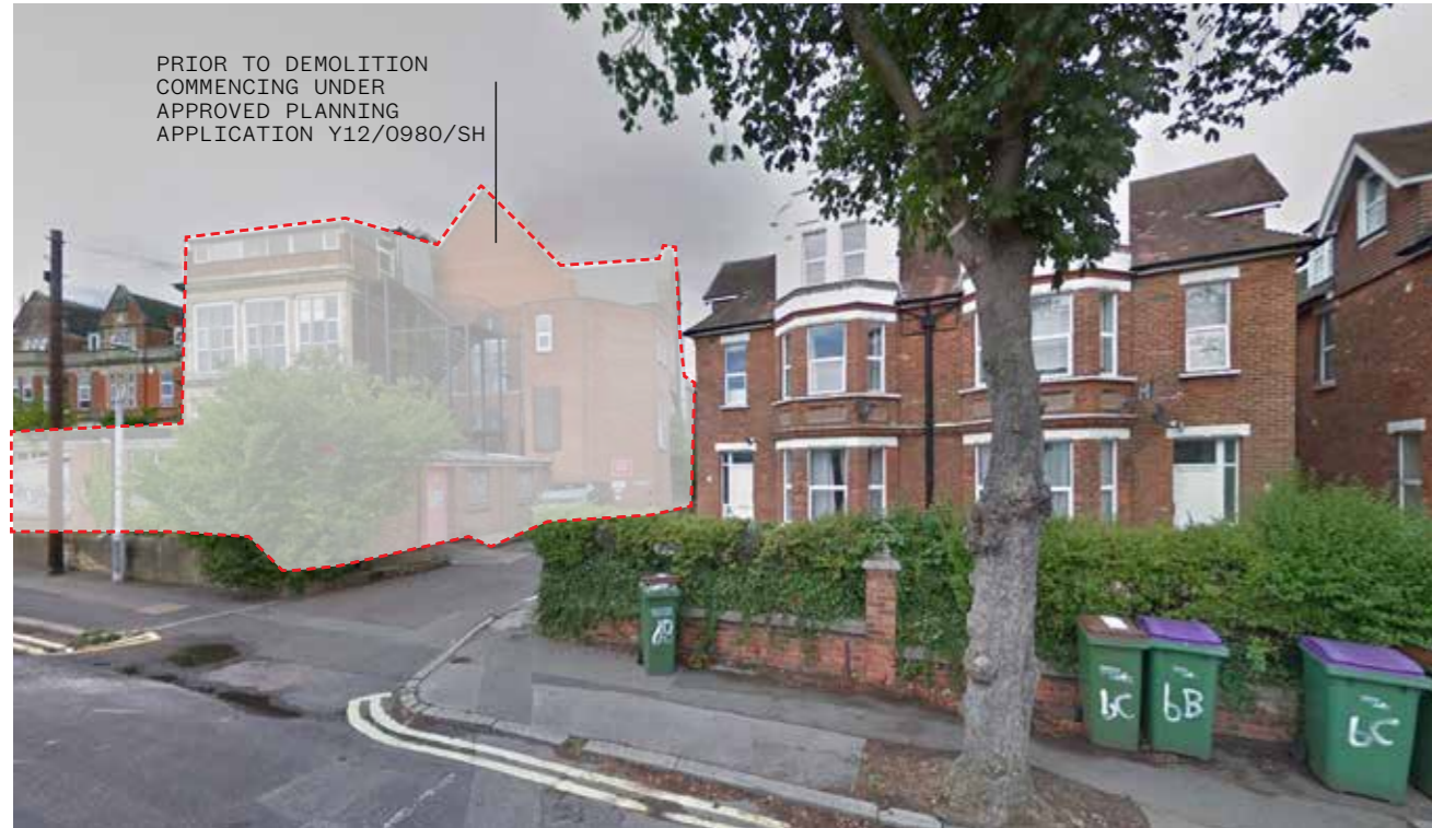
A. View looking at the East Wing of RVH to be demolished and existing access on the east boundary of the site
