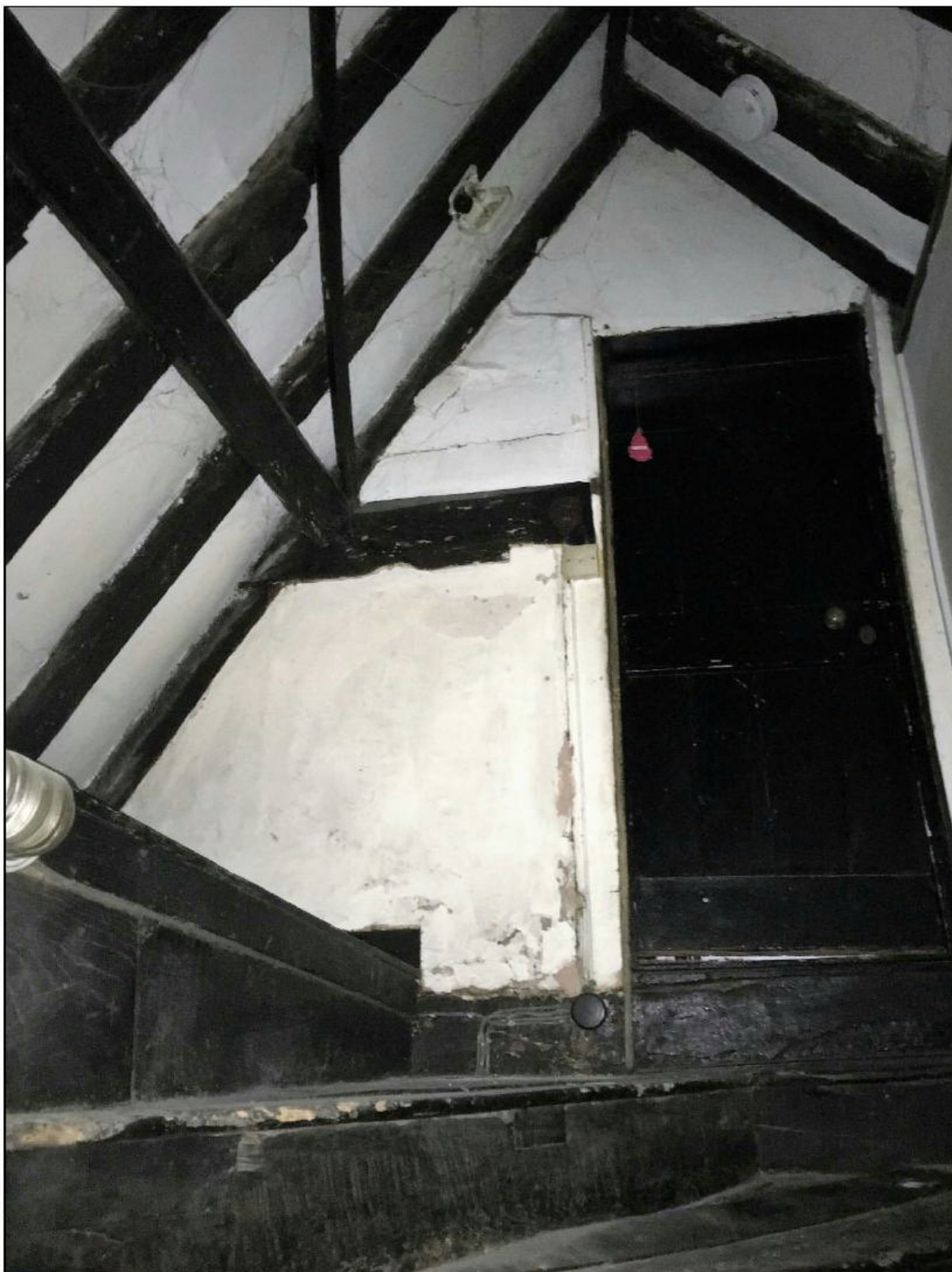
Figure 10: Roof timbers in the historic core of the pub. The presence of a roof plate indicates a late date
