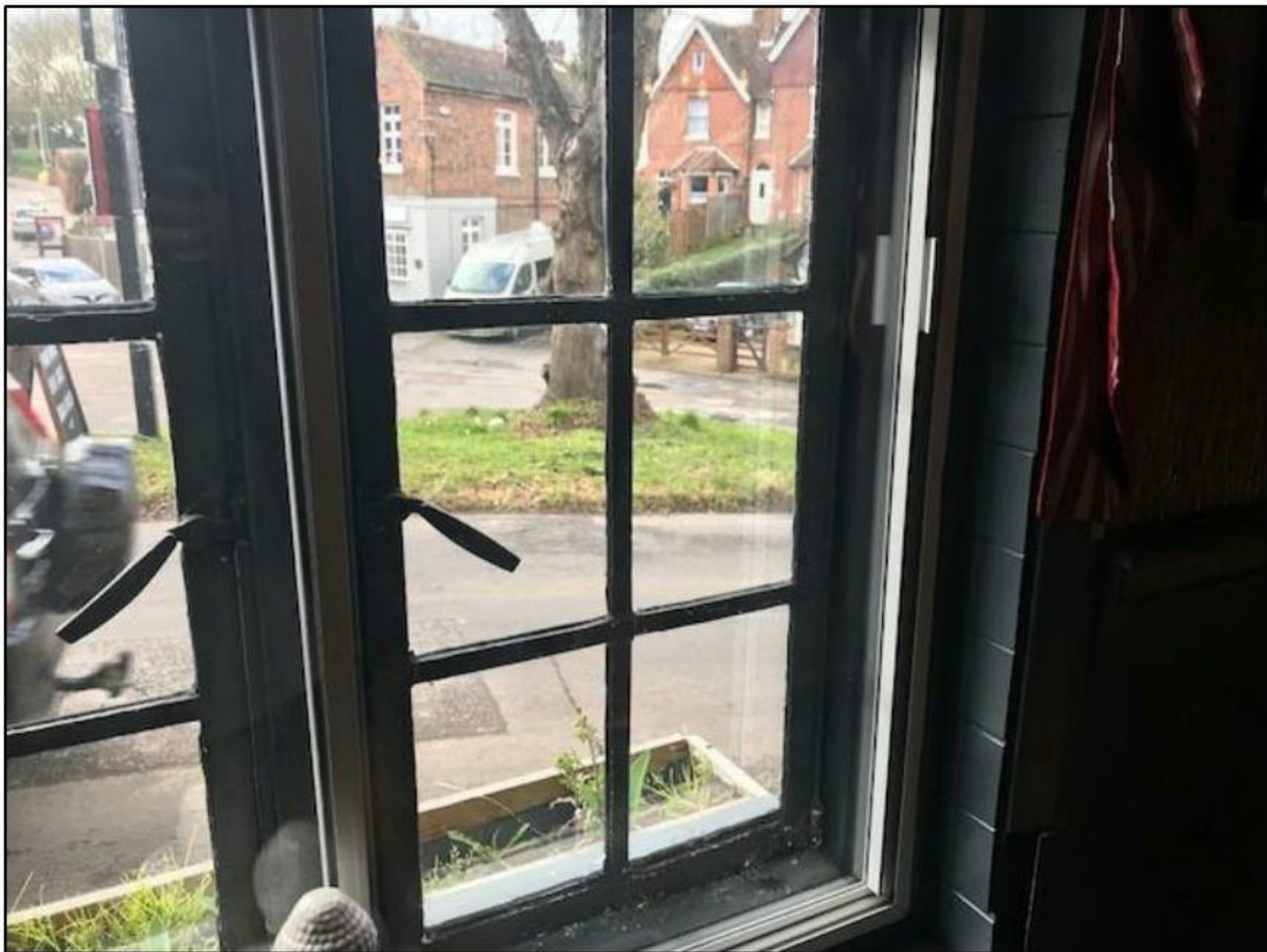
Photograph showing secondary glazing inside public bar
