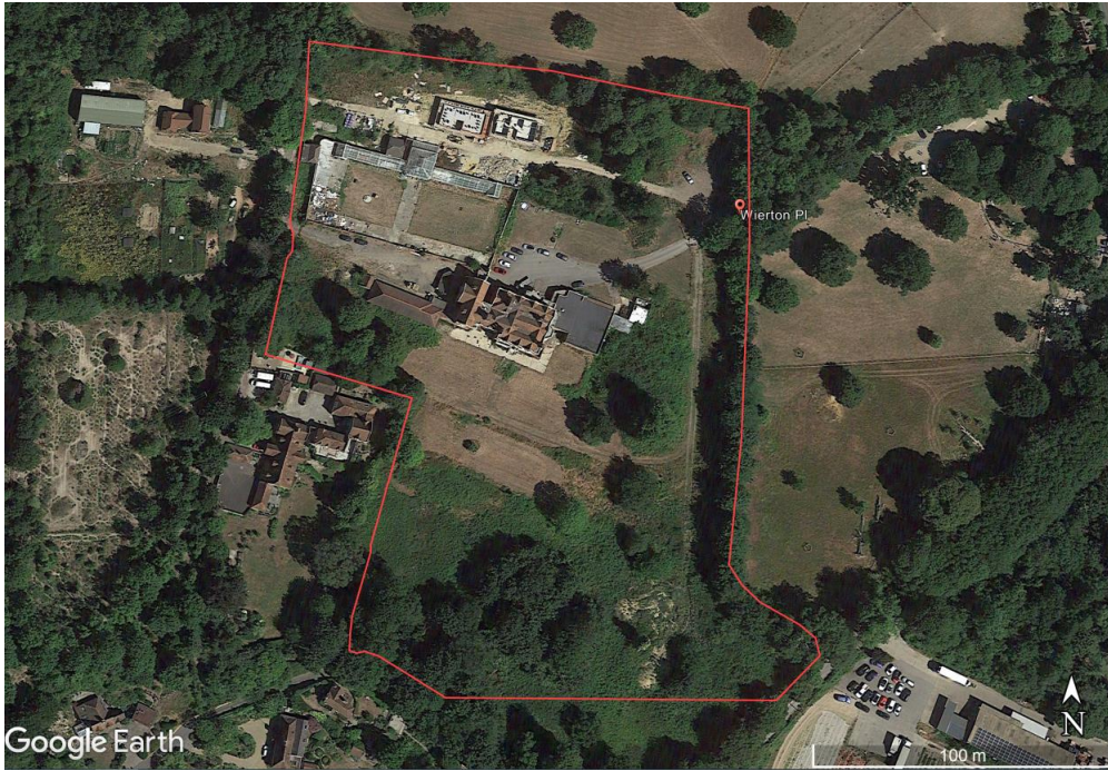
AP 1. View of site 2022 (Google Earth)
