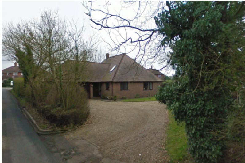
Thorne Lodge- to the east of the application site
