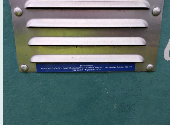
Signage Affixed to an Air Vent On the Eastern Side of the Gas Installation
