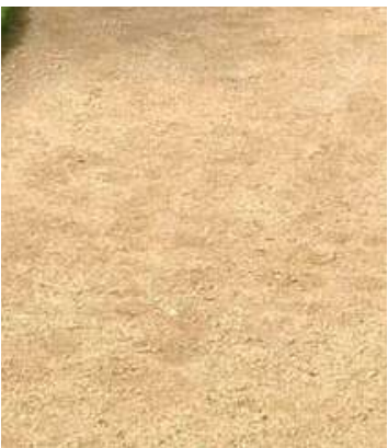
SURFACE TYPE 3 - SELF - BINDING GRAVEL Colour: Buff Locations: Footpaths to public open space
