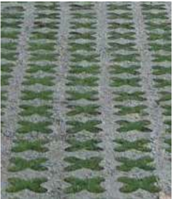
PAVING TYPE 5 - Grasscrete Locations: Emergency access routes
