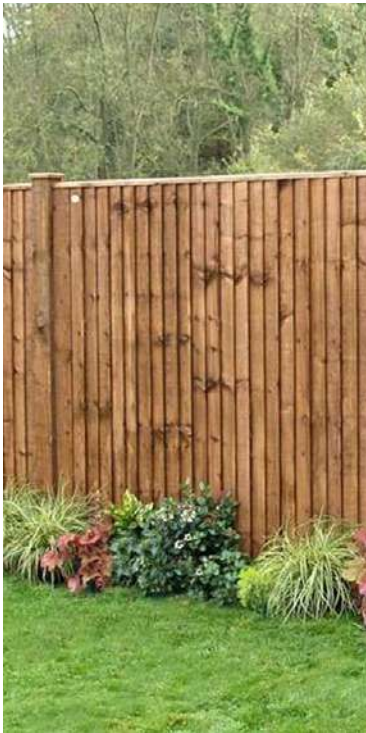
Fencing for residential garden
