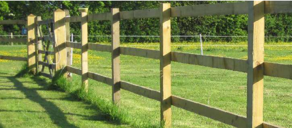
1.5m high timber post and rail fence
