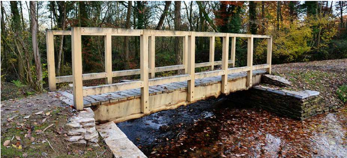
Timber bridge over Iwade Stream
