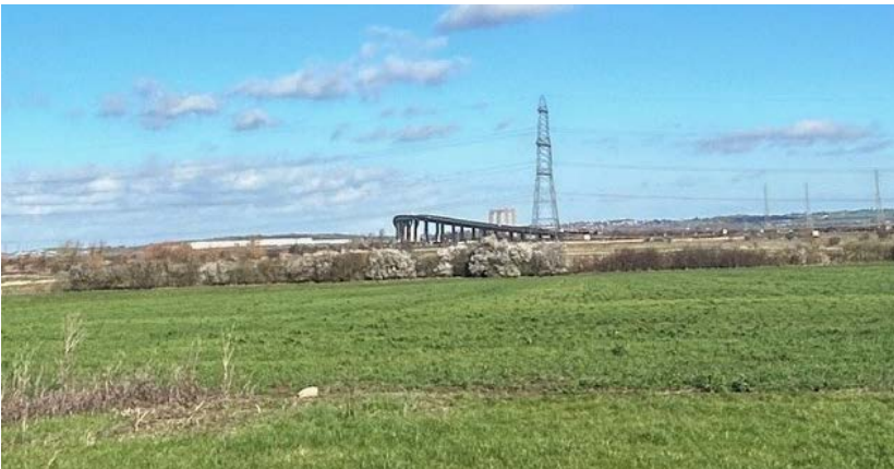
The Sheppey Crossing, seen from the site
