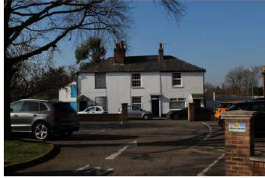
1-5 Bradbourne Road; 2 storey terrace
