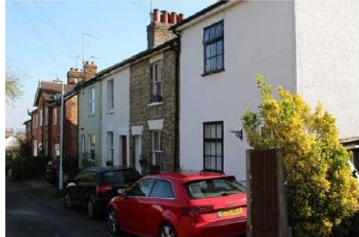
11-14 Bethel Road; 2 storey terrace
