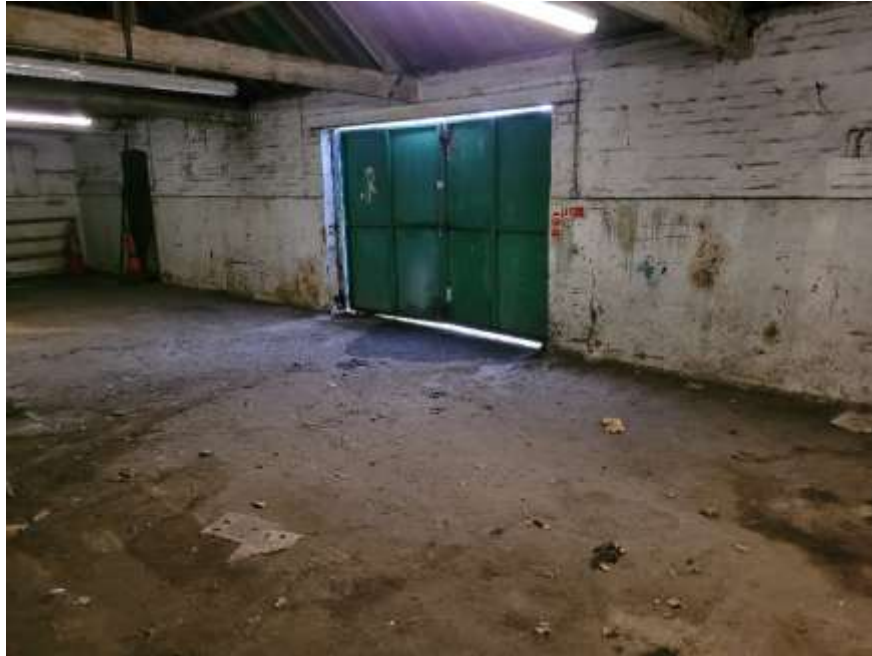
Photo 5 – internal floor area of barns. Concrete in good condition with no visual or olfactory evidence of any staining. Dark patch by doorway is rainwater ingress.
