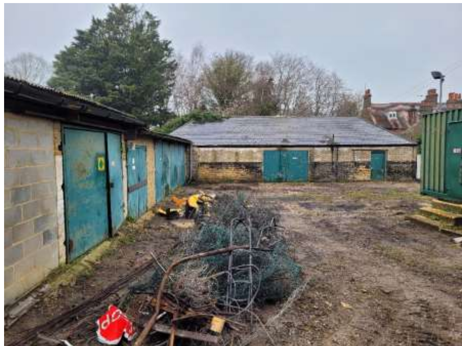
Photo 2 – view north of workshop/storage barns. Suspected ACM roofing on left hand barn in photo. Pile of segregated metal awaiting collection for recycling.
