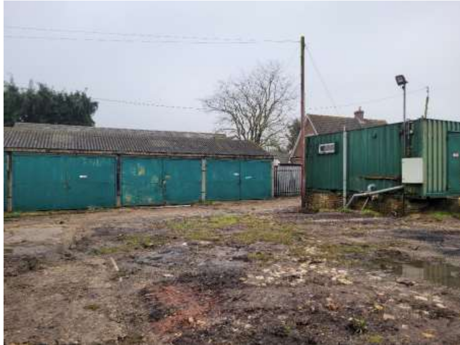
Photo 3 – view east across site, showing another storage barn (with possible ACM roofing) and container used as site office/welfare unit.
