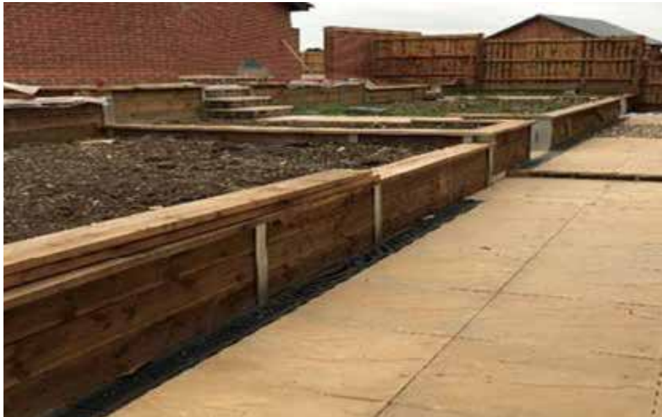
Timber sleeper retaining features in rear gardens
