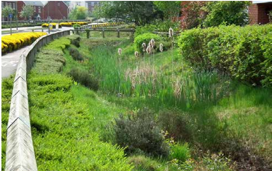
Example of a swale running parallel to the street
