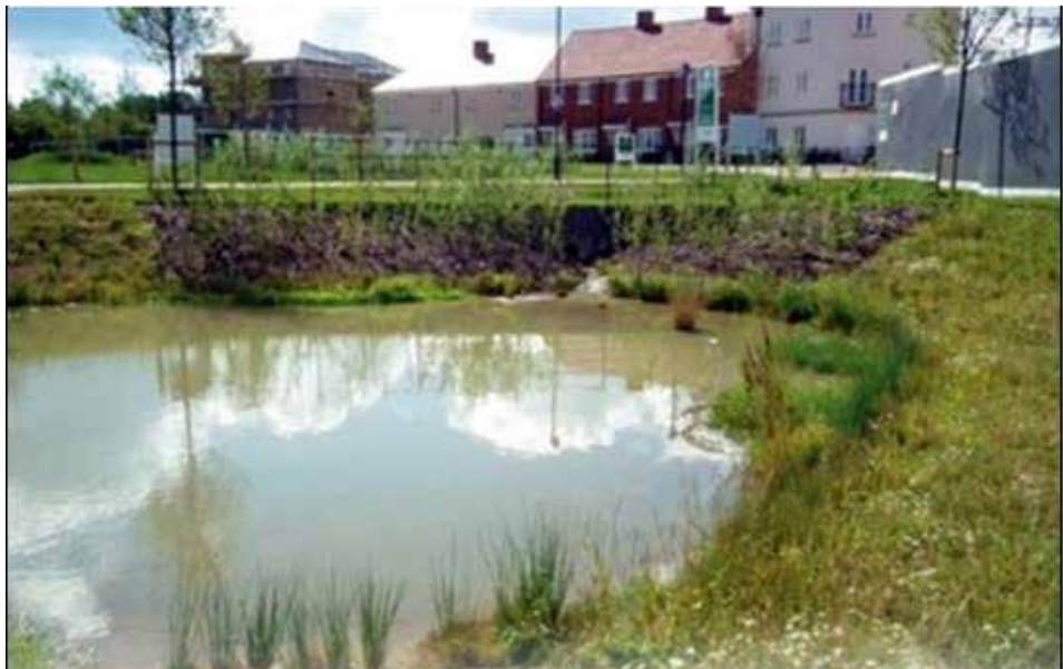
Example of attenuation area with planted edges
