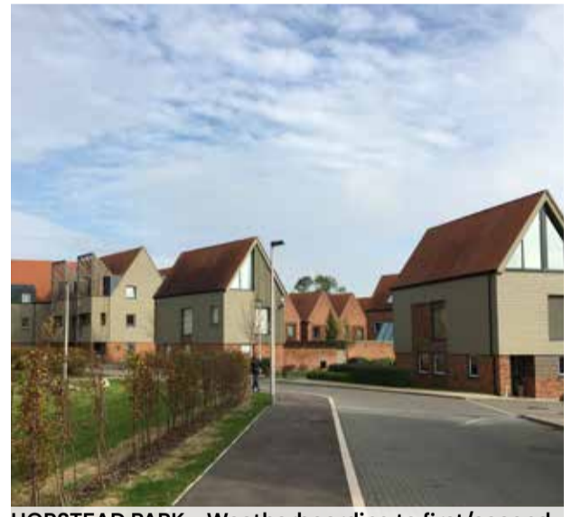
HORSTEAD PARK - Weatherboarding to first/second floor on larger key buildings
