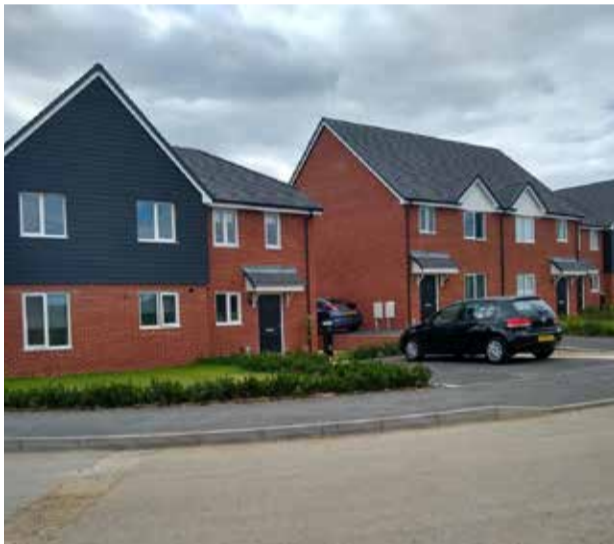
HOO – corner turning dwellings address the street and public open spaces providing natural surveillance
