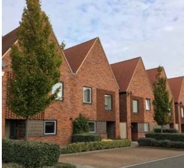
HORSTEAD PARK – Gable fronted units add a scene of rhythm and break up roofscape
