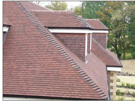
Phalempin Imerys plain clay tiles to main roof colour - Horsham Mix
