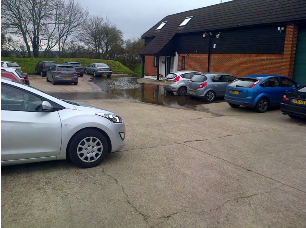
Groundwater flooding of commercial property at Northdown Close. Water unable to discharge through soakaways due to groundwater level. Photo taken on 7 th March 2014. (Source: A. Brauning, KCC)
