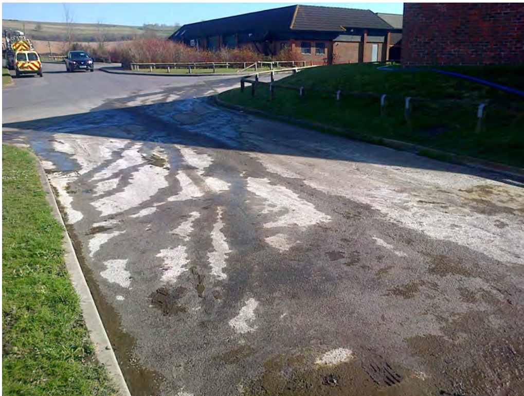
Excess groundwater flows from soakaway being pumped into nearby culvert by landowner to reduce flooding impact. Taken on 20 th March 2014. (Source: A Brauning, KCC)
