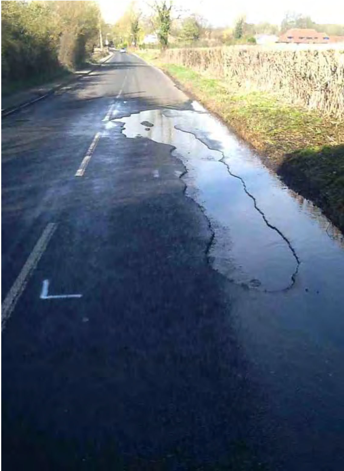
Water issuing from field boundary and from beneath road surface causing damage to road surface. Taken on 20th March 2014. (Source: KCC Highways)
