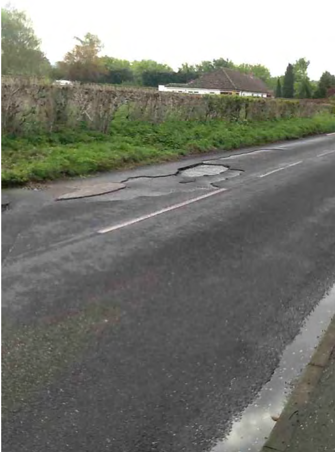
View of lifted road surface at south east boundary of site once groundwater flow had ceased. Photo taken 22 nd April 2014 (Source: KCC Highways)
