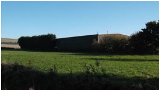
Fig.5 View of Ashmill Business Park from within Site
