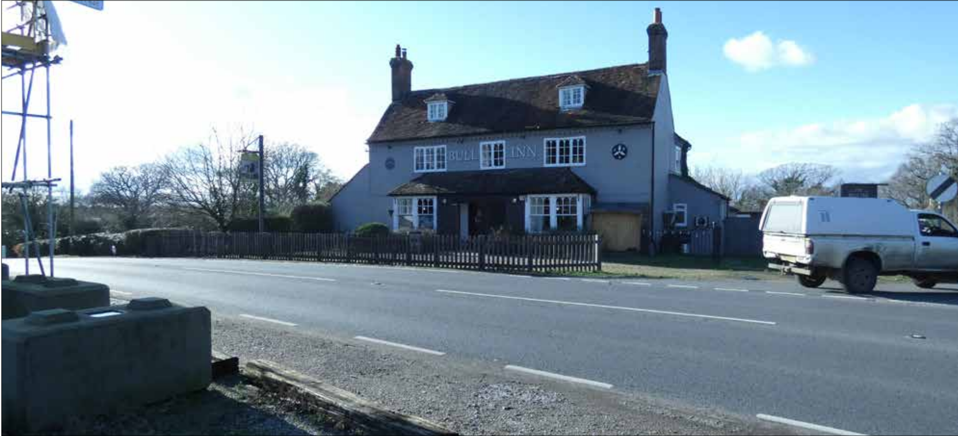
Photo 1: Viewpoint 1 - The Bull Inn, The Stables of Bull Inn, AW277 Public Footpath, A28 Ashford Road
