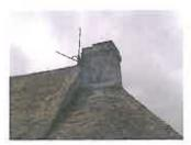
It is clear that the top section of the stack has been rebuilt in previous years and it is more than likely that this will have pre-dated Listing.
