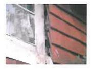
detailing round the rear window at first floor level where bird ingress is occurring. It is likely that the tiles in this area will need to be stripped and re-detailed.
