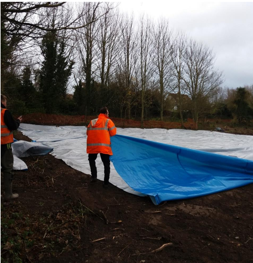
Positioning the stockpile geotextile liner
