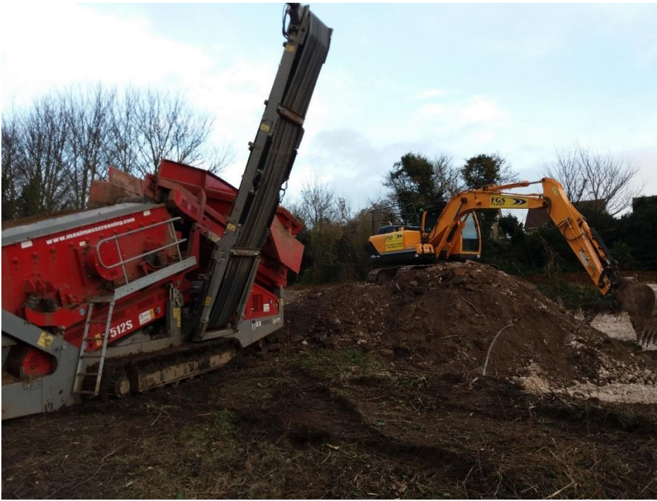
Excavator and Maximus screener in the contaminated area.
