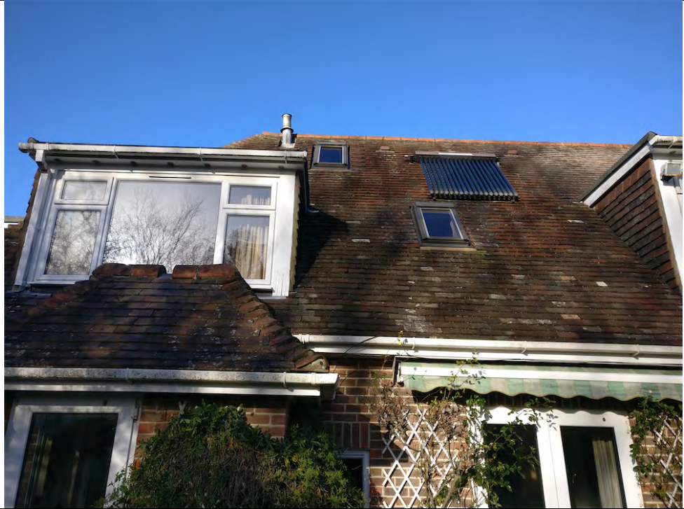
Photograph 5: Rear aspect of the cottage (B2).
