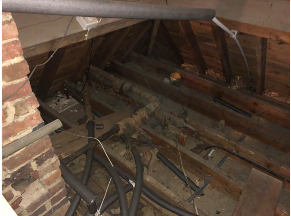
Photograph 3: Western void space within Ashplatts house in which bat droppings were found.
