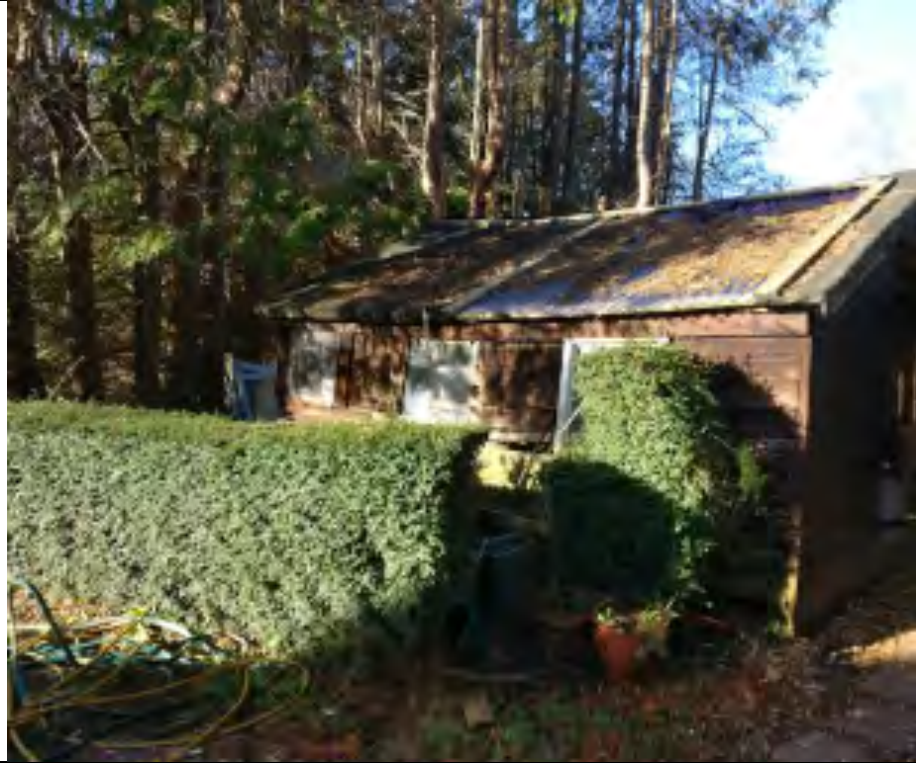
Photograph 9: Shed (B4) showed no potential roost features or signs of roosting bats.
