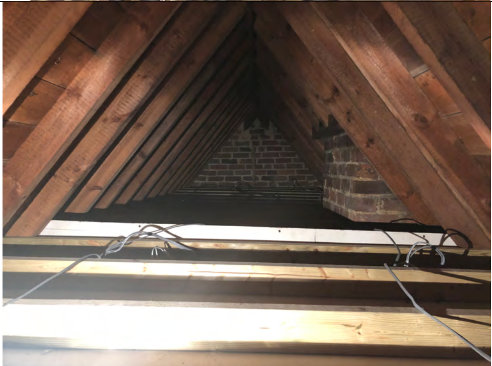
Photograph 4: Void space within Ashplatts house located between roof and dropped ceiling, no evidence of roosting bats observed.
