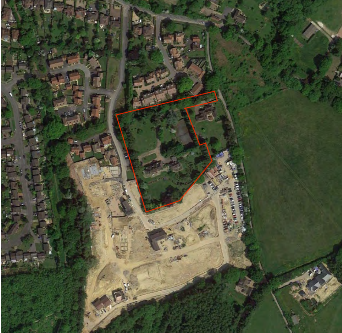
Figure 1: Approximate location of the red line boundary
