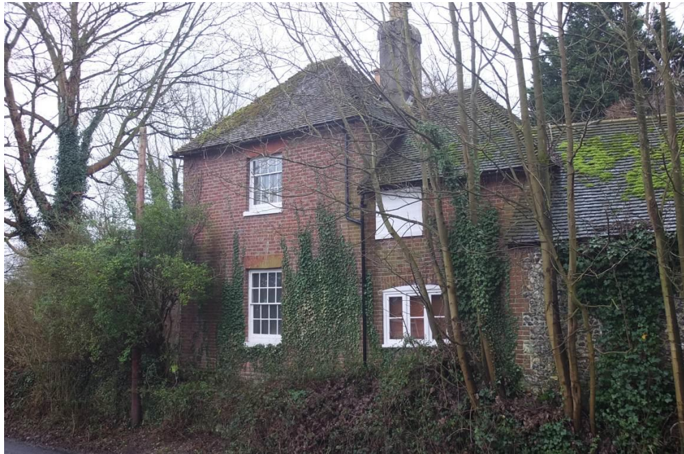
View of house from Maidstone Road.
