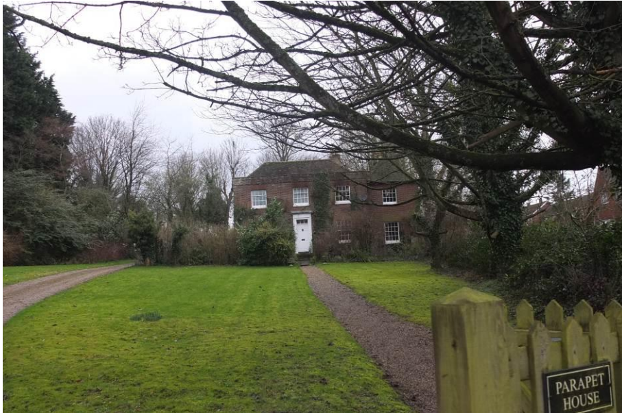
Front View of Parapet House from footpath
