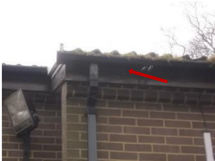
Photograph 19 Eastern elevation of the Multi Agency Services building showing the hole in the fascia board.
