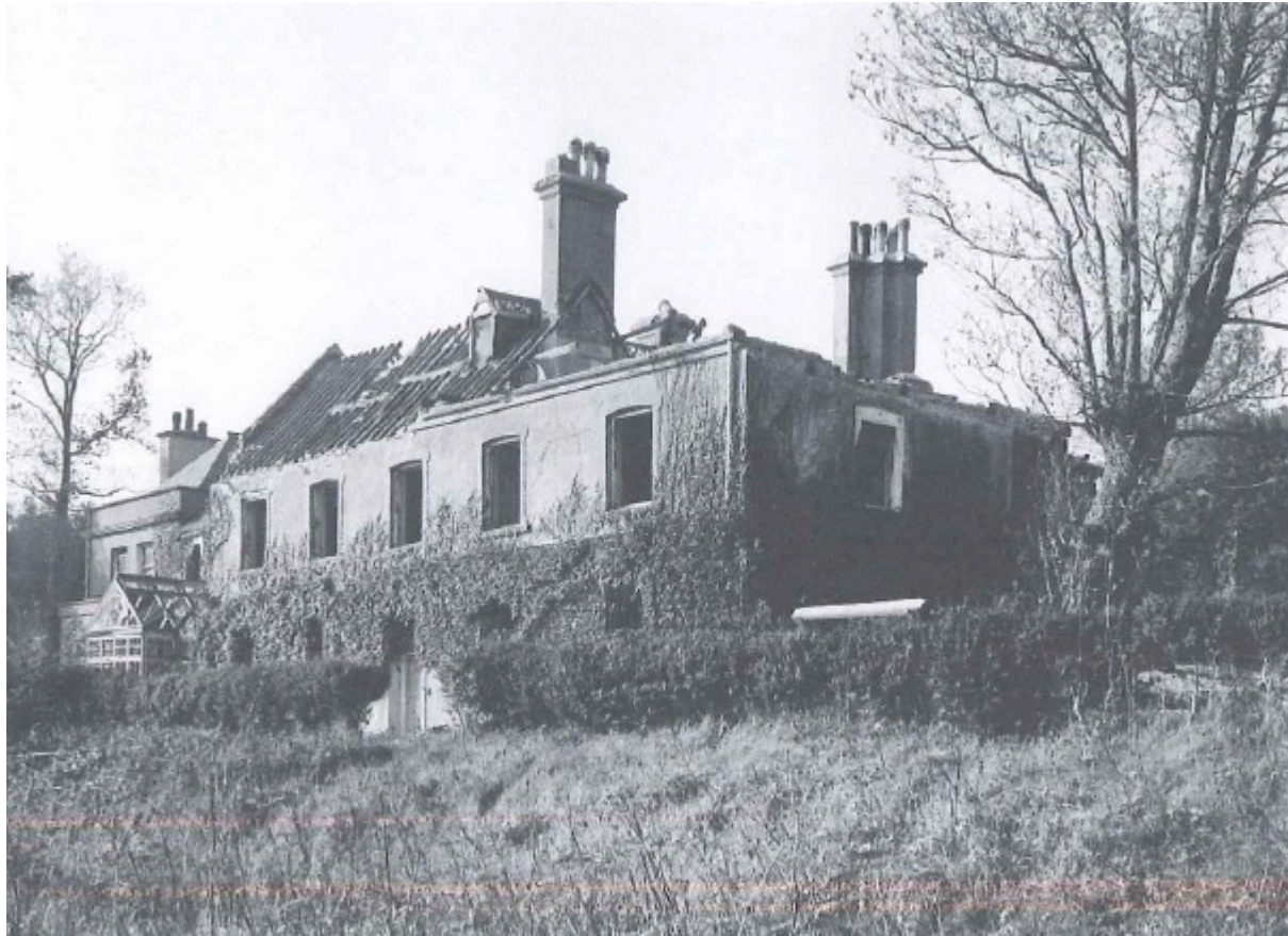
The Grove in ruins. The photograph shows the building on higher ground looking up from the South East.
