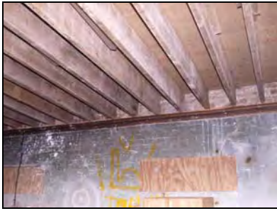
6959-0013 Stable, interior, ground floor, blocked windows on the north elevation. Facing north
