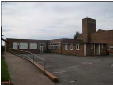
6959-0034 Main school building, eastern elevation and far east end of the northern elevation. Facing southwest
