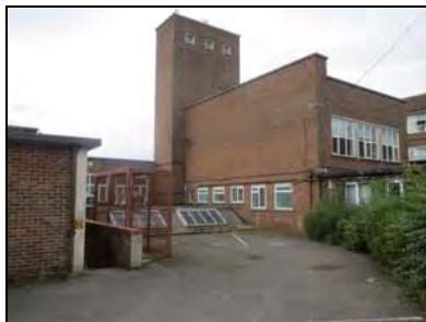
6959-0035 Main school building, eastern end of the northern elevation. Facing southwest
