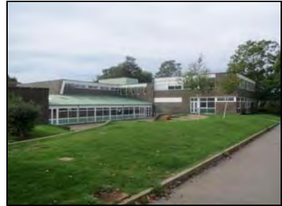
6959-0042 Main school building, western end of the northern elevation. Facing west
