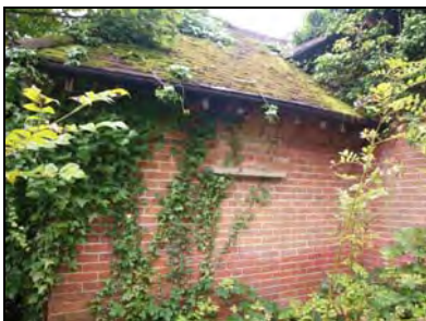
6959-0022 Stable, northern elevation of the far eastern projection. Facing southwest
