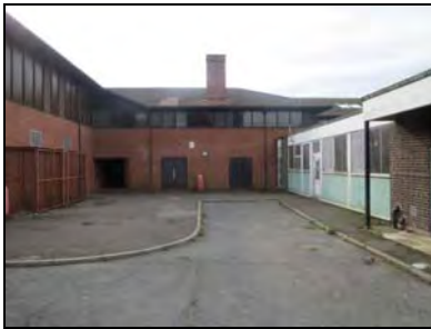
6959-0044 Main school building, 'L' shaped recess leading to the lower partially enclosed courtyard, western end of the northern elevation. Facing south
