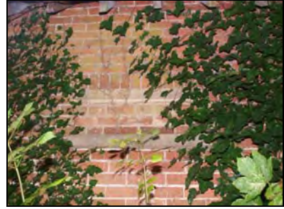
6959-0027 Stable, northern elevation, detail of blocked window. Facing south
