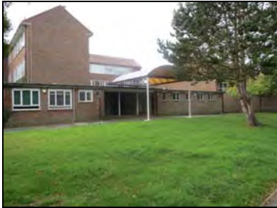
6959-0040 Main school building, reception entrance, central section of the northern elevation. Facing southwest
