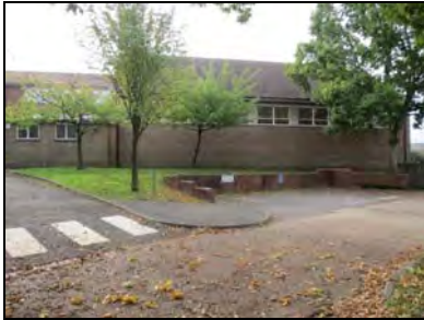
6959-0041 Main school building, central section of the northern elevation. Facing southwest
