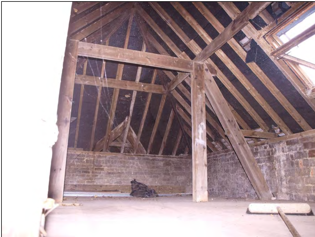
Plate 3.16 Stable, interior, first floor, detail of roof composition, facing east (6959-0008)
