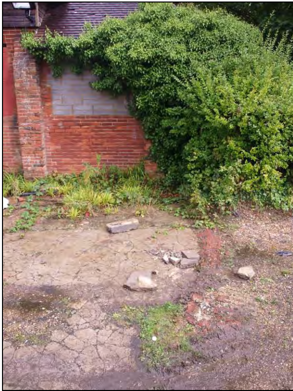
Plate 3.17 Stable, far eastern end of southern elevation and brick footings in southern courtyard, facing north (6959-0020)
