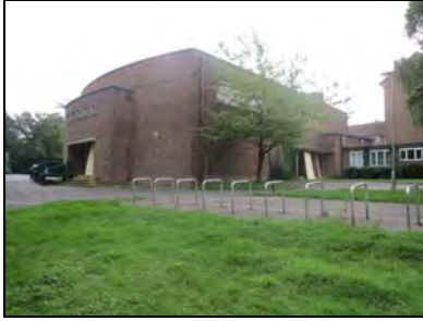
6959-0038 Main school building, eastern projection located on the northern elevation. Facing south
