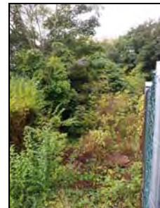
6959-0021 Stable, northern elevation, restricted access due to dense vegetation. Facing west
