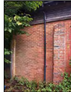
6959-0018 Stable, far western end of the southern elevation. Facing northwest
