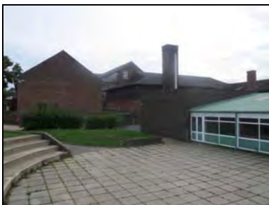
6959-0047 Main school building, western end of the northern elevation, facing the entrance to the 'L' shaped recess. Facing east
