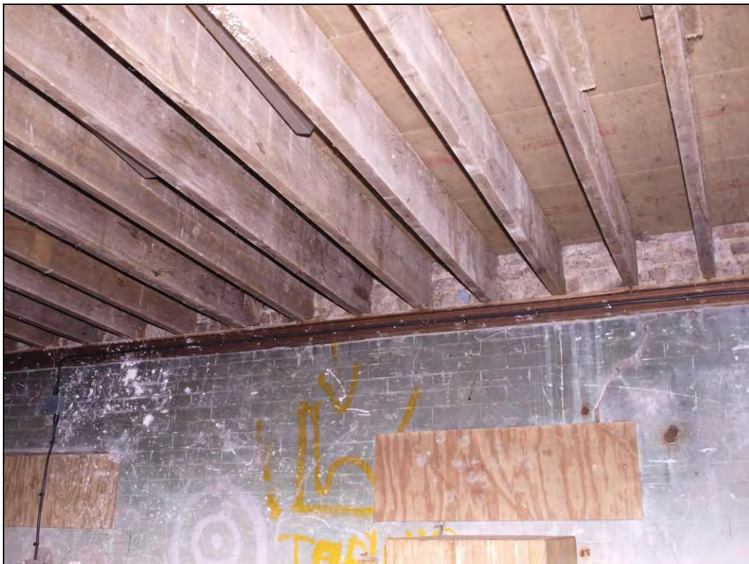
Plate 3.14 Stable, interior, ground floor, blocked windows on the north elevation, facing north (6959-0013)
