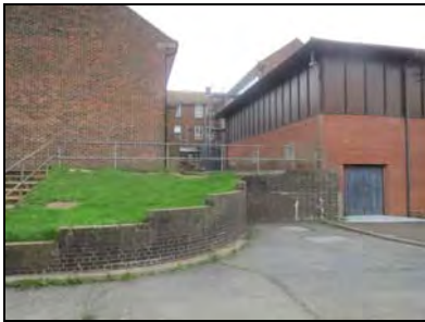
6959-0043 Main school building, 'L' shaped recess leading to an elevated partially enclosed courtyard, western end of the northern elevation. Facing east
