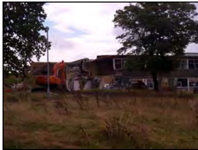
6959-0032 Main school building, northern and western elevations, under demolition. Facing east
