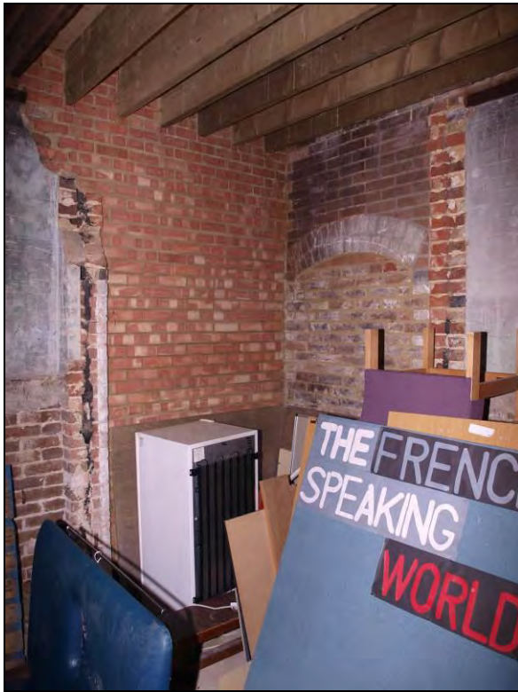
Plate 3.13 Stable, interior, ground floor, detail of southwest corner alterations, facing southwest (6959-0006)
