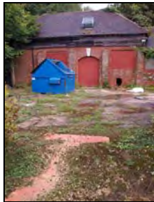
6959-0031 Stable, southern elevation, detail of concrete and tile hardstanding of the southern courtyard. Facing north
