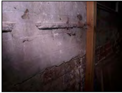
6959-0014 Stable, interior, ground floor, detail of rendered brickwork on the southern elevation. Facing southwest
