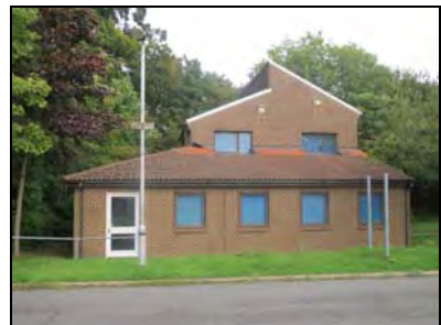
6959-0036 School building complex, detached building located in the far northeast corner of the site. Facing north
