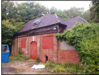
6959-0017 Stable, southern and eastern elevations. Facing northwest
