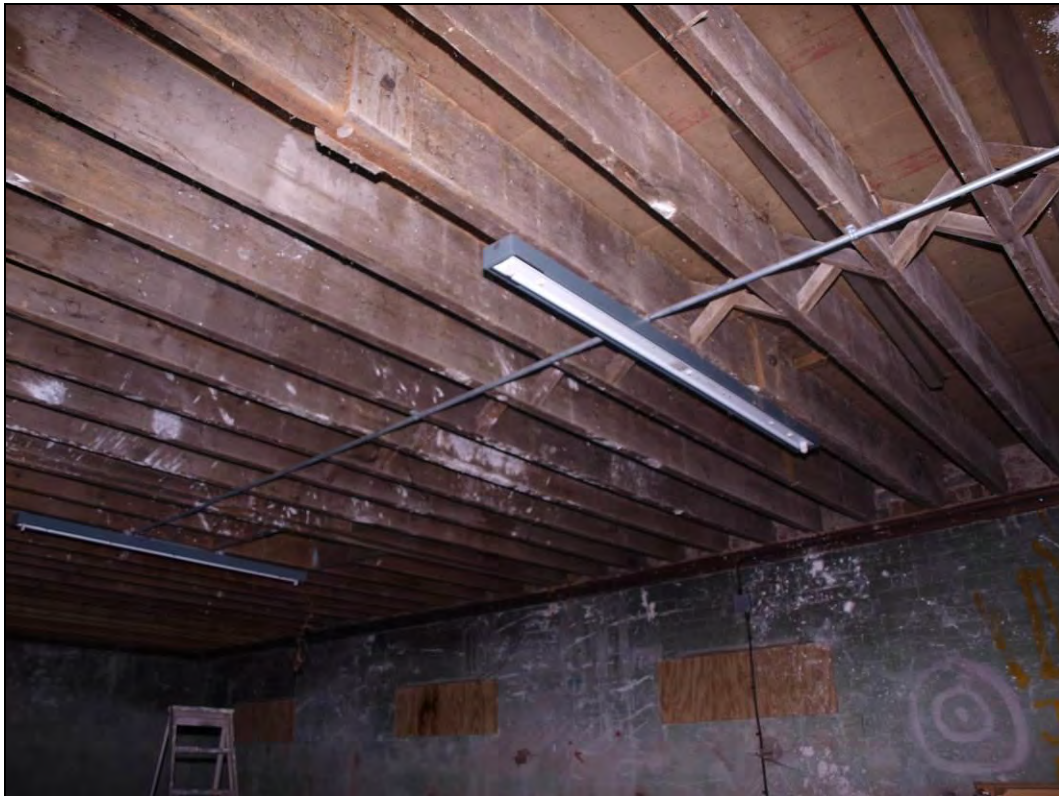
Plate 3.15 Stable, interior, underside of first level flooring, facing northwest (6959-0002)
