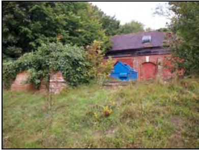
6959-0028 Stable, southern elevation and detail of boundary brick wall enclosing the southern courtyard. Facing north
