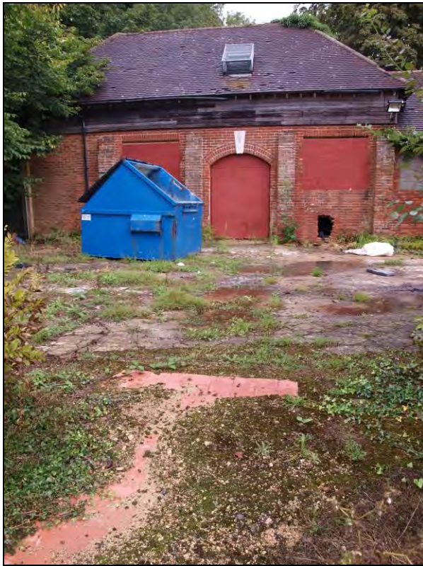
Plate 3.19 Stable, southern elevation, detail of concrete and tile hardstanding of the southern courtyard, facing north (6959-0031)
