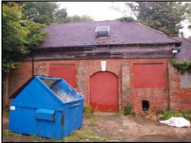
6959-0016 Stable, southern elevation. Facing north
