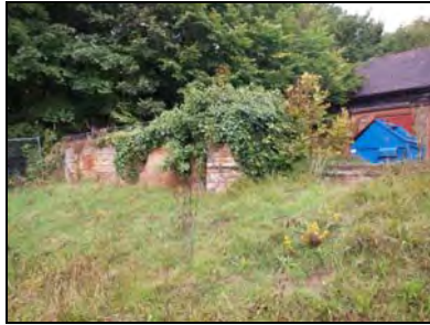
6959-0029 Detail of boundary brick wall enclosing the southern courtyard. Facing northwest
