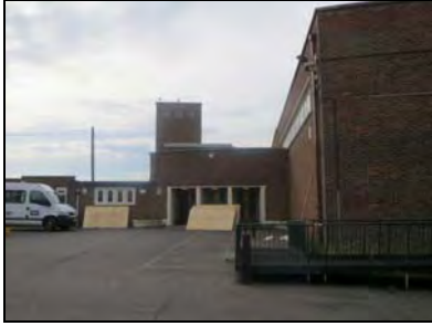
6959-0037 Main school building, eastern end of the northern elevation. Facing south
