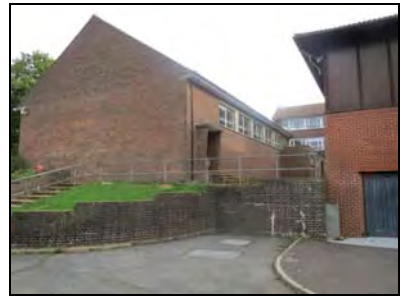
6959-0045 Main school building, 'L' shaped recess leading to an elevated partially enclosed courtyard, western end of the northern elevation. Facing northeast
