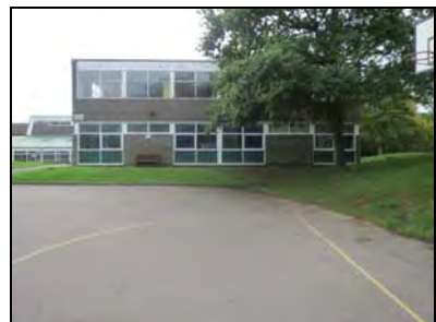
6959-0048 Main school building, far western end of the northern elevation. Facing south
