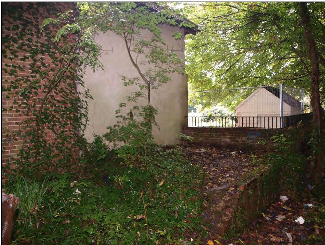
Plate 3.18 Stable, western elevation and raised platform, facing southeast (6959-0026)
