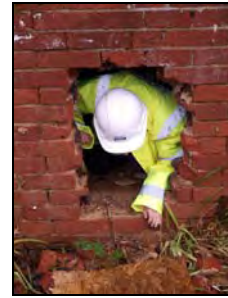
6959-0015 Stable, southern elevation, interior access at the eastern end. Facing north
