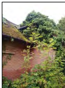
6959-0023 Stable, northern elevation of outshut, east elevation of main building. Facing southwest
