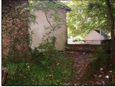
6959-0026 Stable, western elevation and raised platform. Facing southeast
