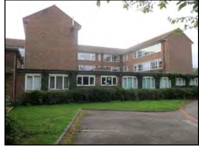
6959-0039 Main school building, central section of the northern elevation. Facing south
