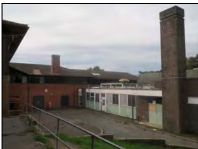
6959-0046 Main school building, taken from the elevated 'L' shaped courtyard facing the lower level courtyard, western end of the northern elevation. Facing southwest
