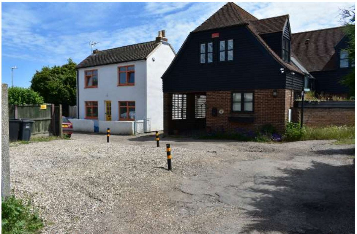
The Old Forge and its neighbour, to the north, Forge Cottage
