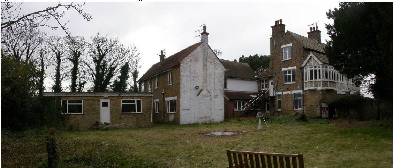
Figure 6: Northern and Eastern elevation of the residential building showing flat roofed single storey extension
