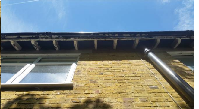
Figure 6: Eaves extending beyond the wall
