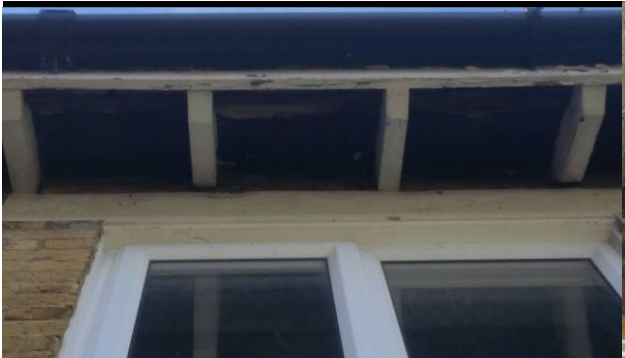
Figure 13: Gap within felt underlining at eaves
