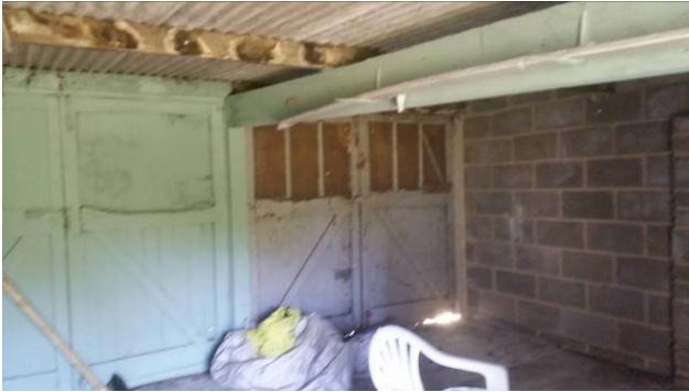
Figure 11: Internal space of outbuilding
