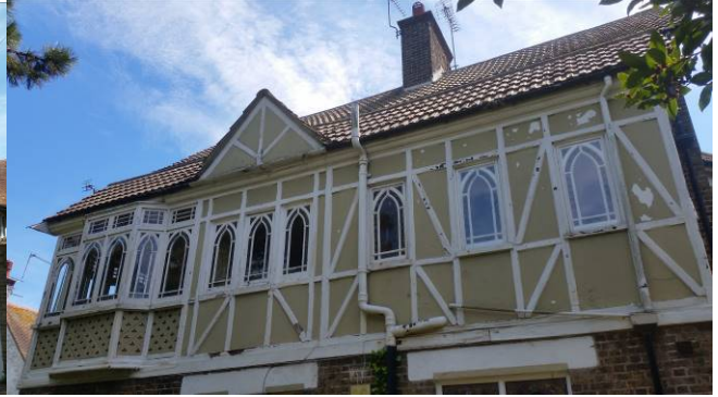
Figure 2: Northern elevation of the main building
