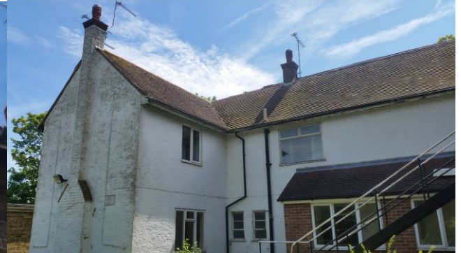
Figure 4: Northern elevation of modern two storey extension
