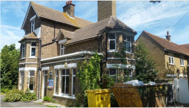
Figure 1: Southern elevation of main building
