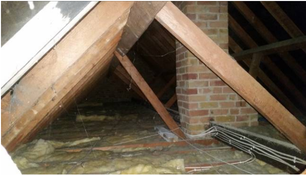
Figure 9: Internal spaces of roof void 4
