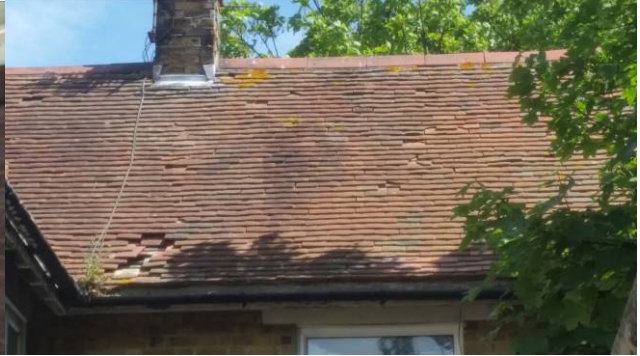
Figure 12: Gaps located beneath missing tiles
