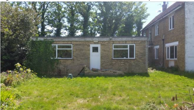
Figure 7: Northern ele. of the single storey flat roof extension
