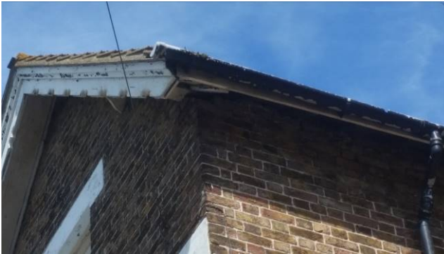
Figure 3: Areas of open eave and soffit within eastern gable end
