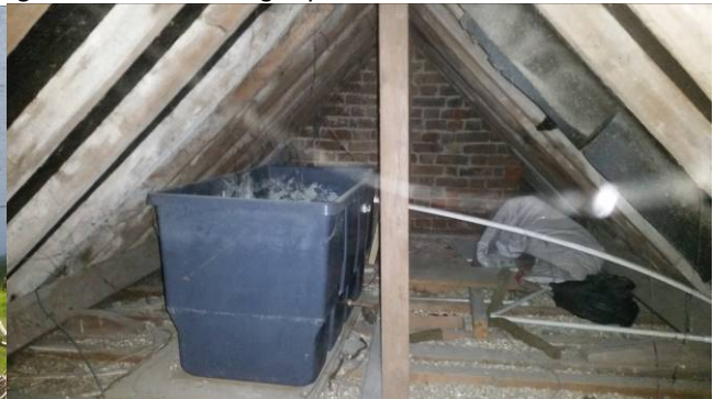
Figure 8: Internal spaces of roof void 1
