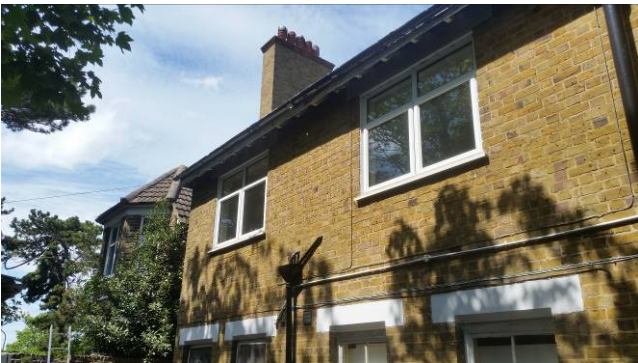
Figure 5: Southern elevation of modern two storey extension
