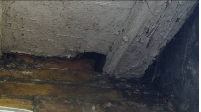
Figure 14: Gap located within soffit on eastern ele. of building
