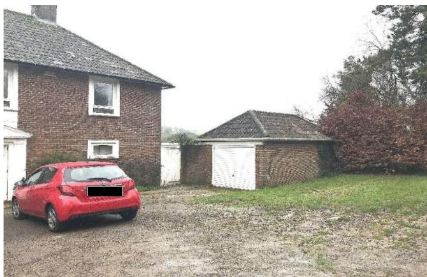
Garage to be demolished.
