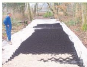
CellWeb during installation
