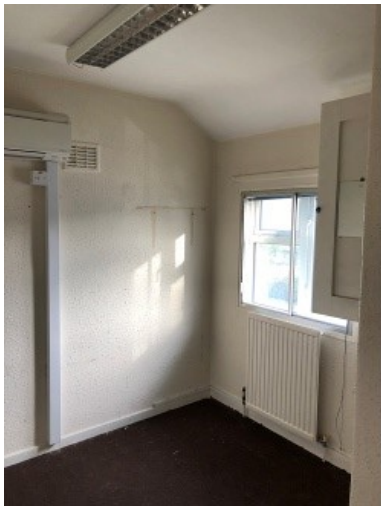
1st floor bedroom 3
