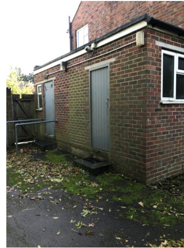
RHS outside stores
