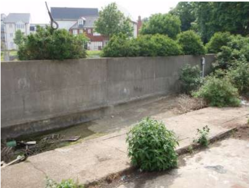
Eastern boundary of site showing extent of flood defence.
