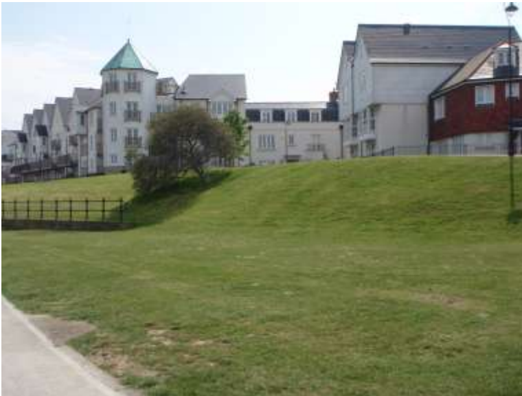
Looking east along flood defence bund in Ingress Park.
