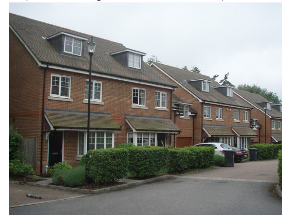
Properties Backing onto northern boundary of Site
