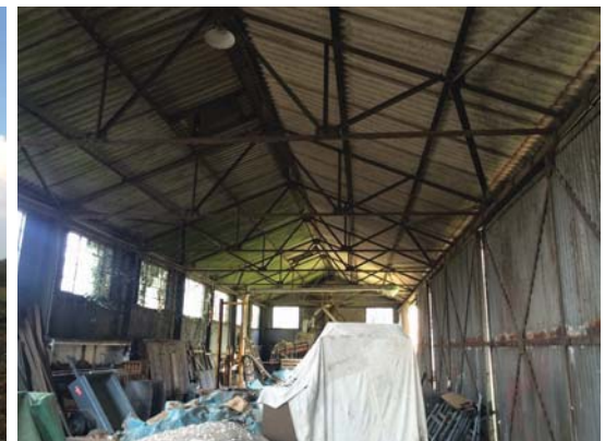
Interior of building B4
