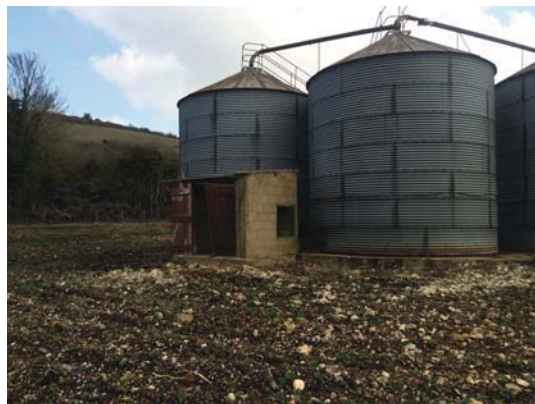
Building B2 (adjacent to silos)
