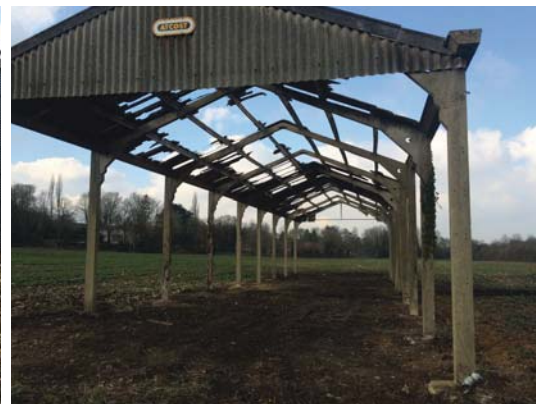
Frame of building B3
