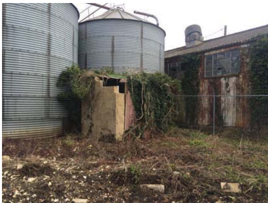
Building B1 (adjacent to silos)
