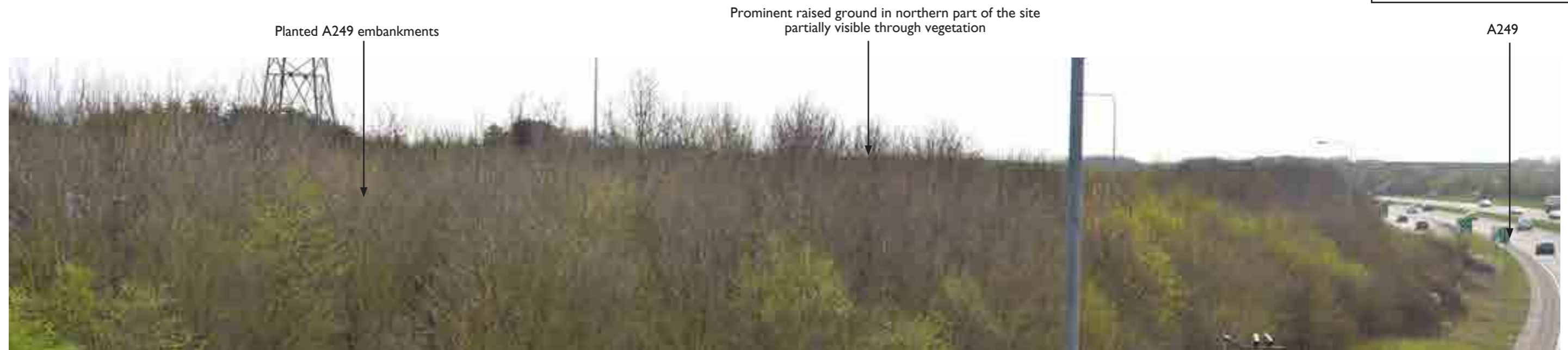
VIEW 10 View from B2005 bridge over A249, south of Iwade, looking south towards the site
