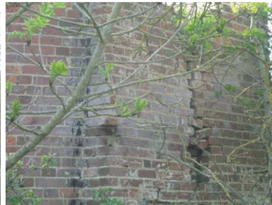
Building B4 - abandoned roundel with cracks in brick work
