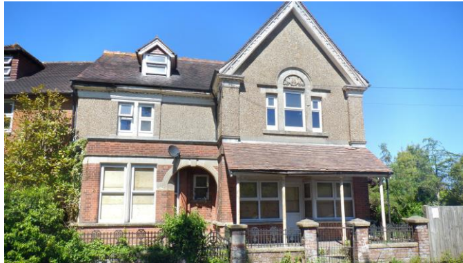
Figure 3: THE FRONT (SOUTH) SIDE OF SECTION A, THE ORIGINAL HOUSE.
