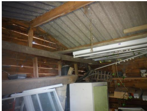
Figure 10: INSIDE THE WOODEN SHED; NOT SUITABLE AS BAT HABITAT.
