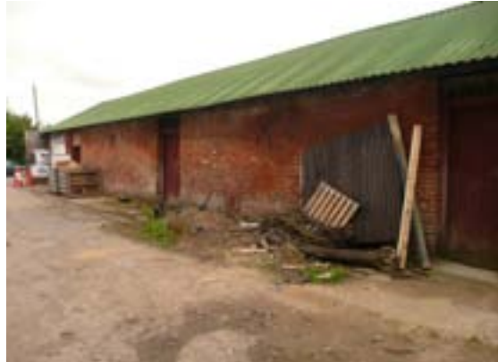
Image 2: Building at centre of brownfield area, running north to south.
