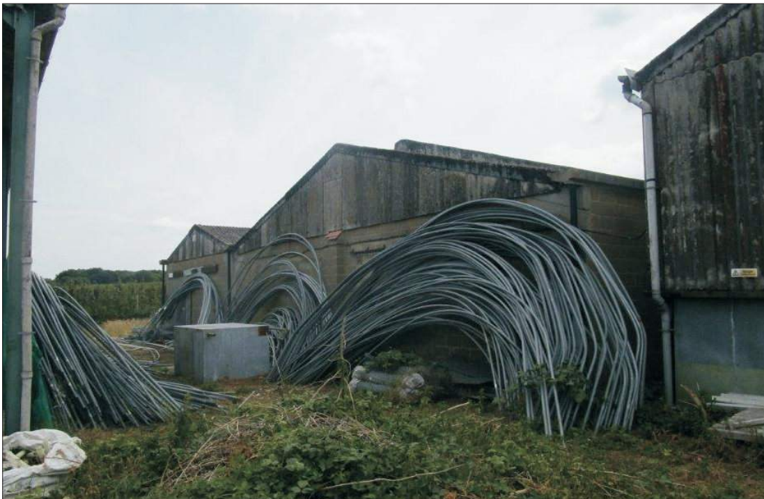
PHOTOGRAPH 2: Building B1 and Associated Recolonising Ground
