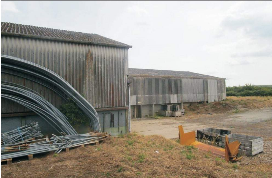
PHOTOGRAPH 3: Building B2 with associated Hardstanding and Recolonising Ground
