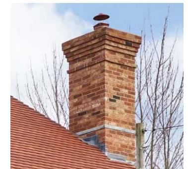
D Brick Chimneys
