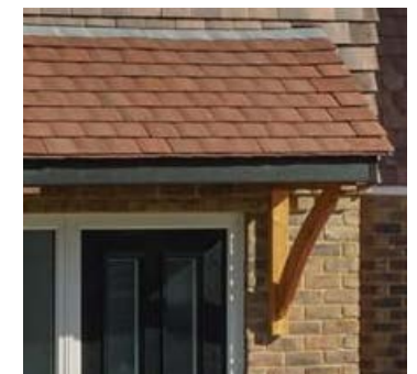
J Timber brackets and detailing
