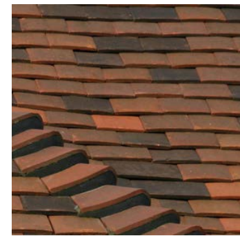
B Dark clay tile roofing
