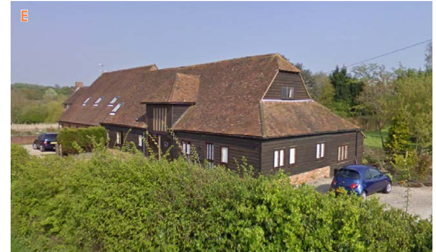
Grade II listed Old Barn with black boarding and large windows, characteristic of the edge of Bethersden.
