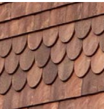
Clay tile hanging with detailing
