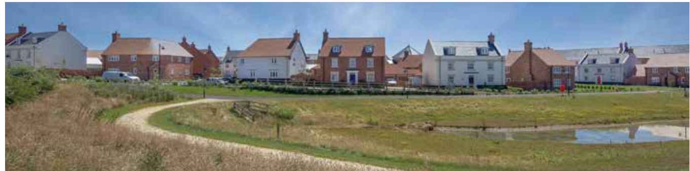
Surface water attenuation pond
