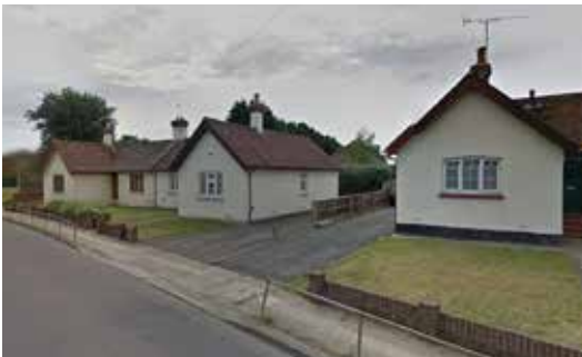
Kiln Barn Road west : Bungalows
