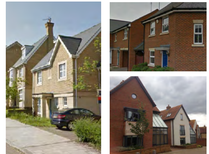
Figure 5.8: Sample of buildings and roofs appropriate for the site
